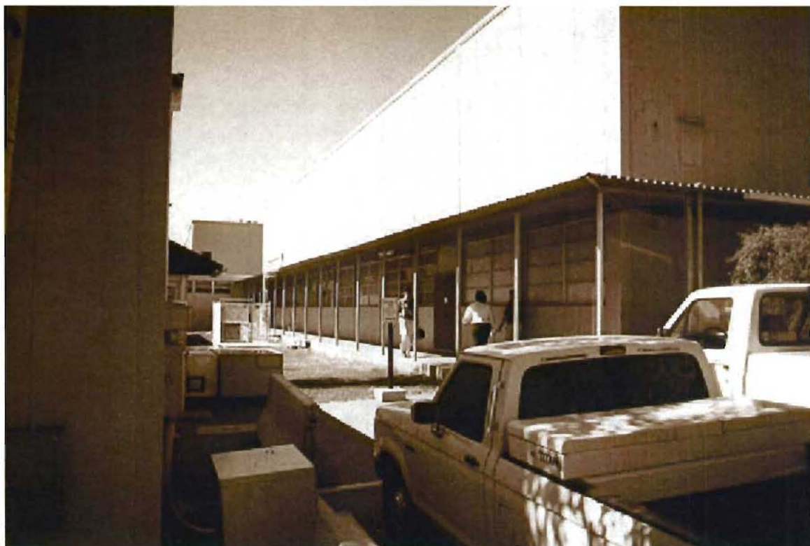
Sherwood Building, TA-3-105, east side, direction southwest
