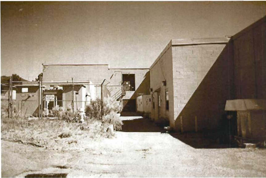
Sherwood Building, TA-3-105, south side, direction north
