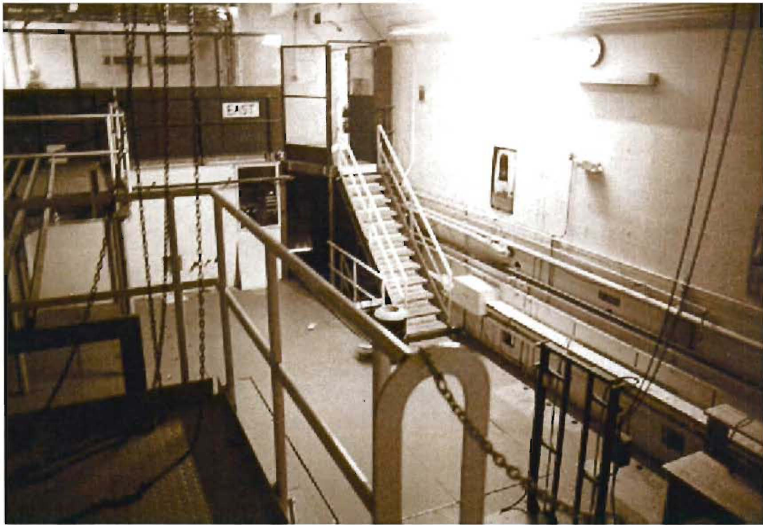
Sherwood Building, TA-3-105, "the pit", mezzanine 1, direction southeast
