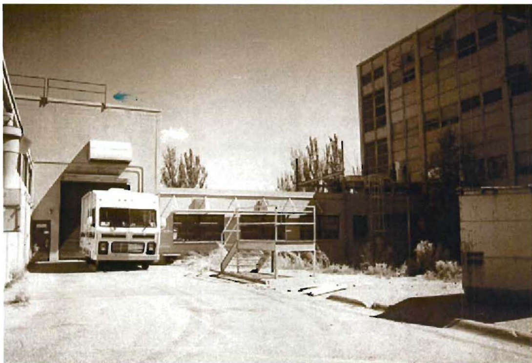
Sherwood Building, TA-3-105, south side, direction north
