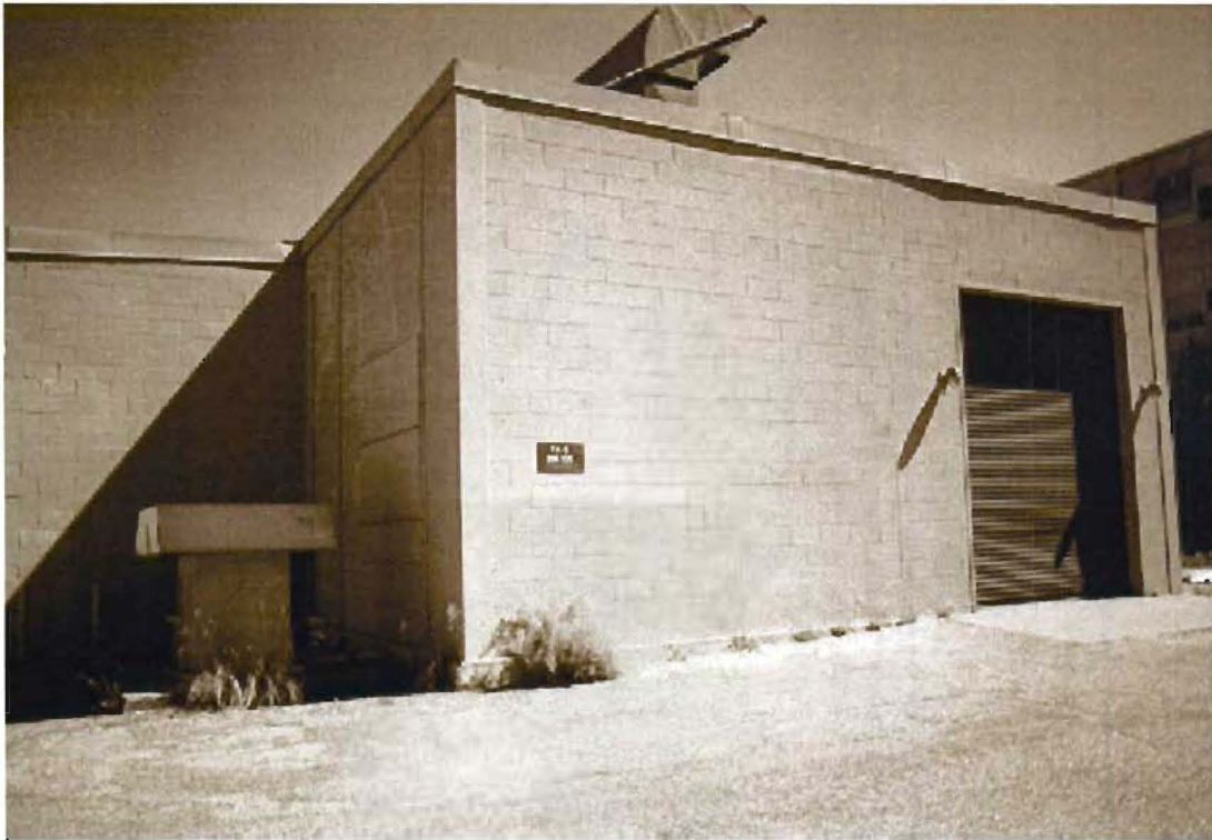
Sherwood Building, TA-3-105, south side, direction north northeast
