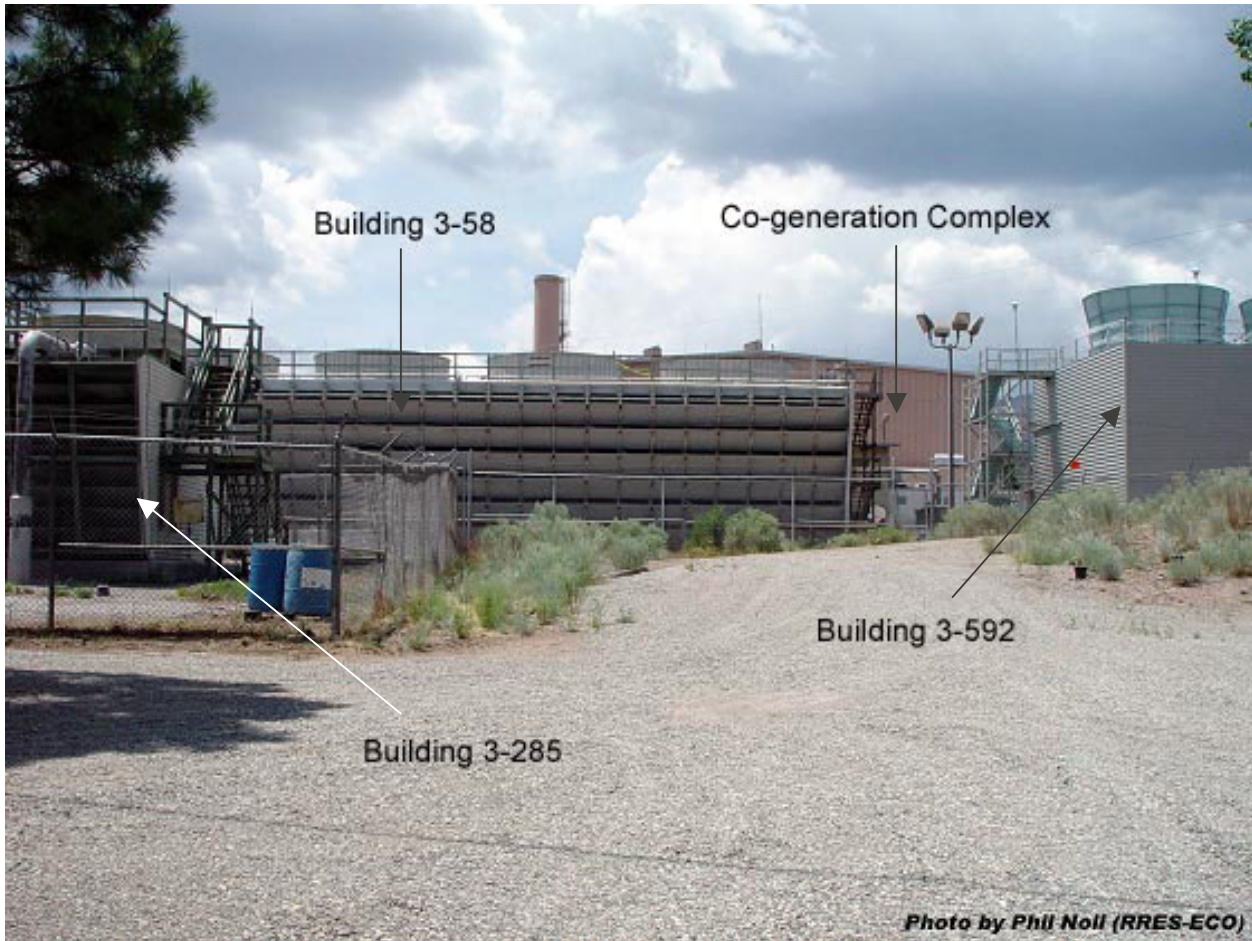
Figure 3. Structures to be demolished and existing Co-generation Complex at TA-3.
