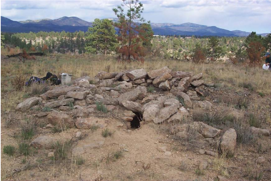
Figure 9.7. LA 12657C, a fire-impacted one- to three-room structure (note the stump hole in the foreground of the photograph).
