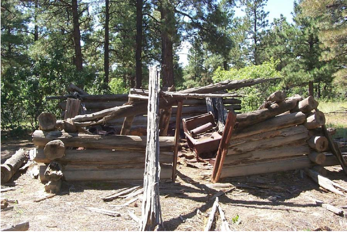
Figure 11.1. LA 21334, the Montoya cabin on Two-Mile Mesa before the Cerro Grande Fire.
