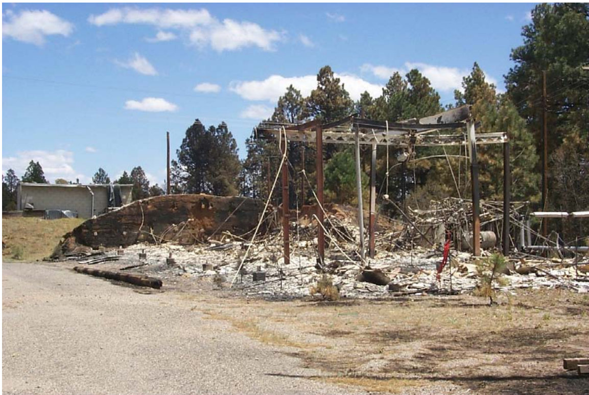
Figure 11.12. TA-16-515 after the Cerro Grande Fire.
