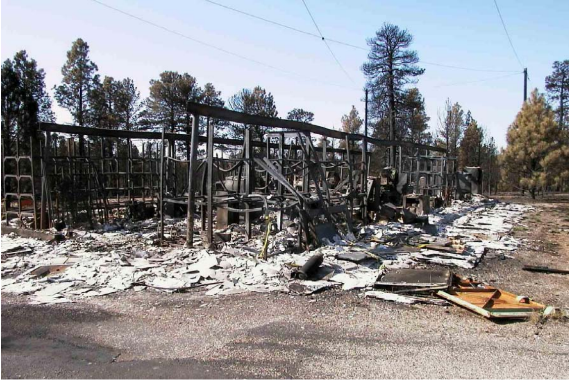
Figure 11.14. TA-40-73 after the Cerro Grande Fire.
