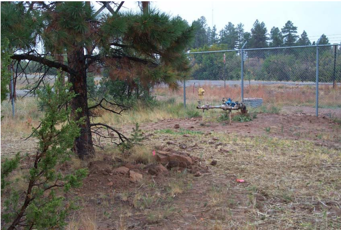
Figure 9.11. LA 137755, a one- to three-room structure impacted by a low-level burn, the partially burned tree in the center of the fieldhouse poses a threat to the site's integrity.
