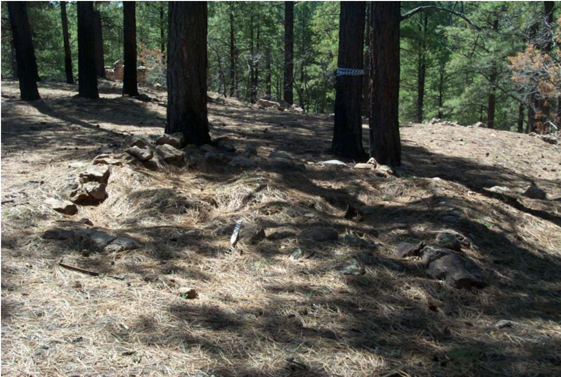
Figure 12.4. LA 86643, the cabin foundation after the Cerro Grande Fire.
