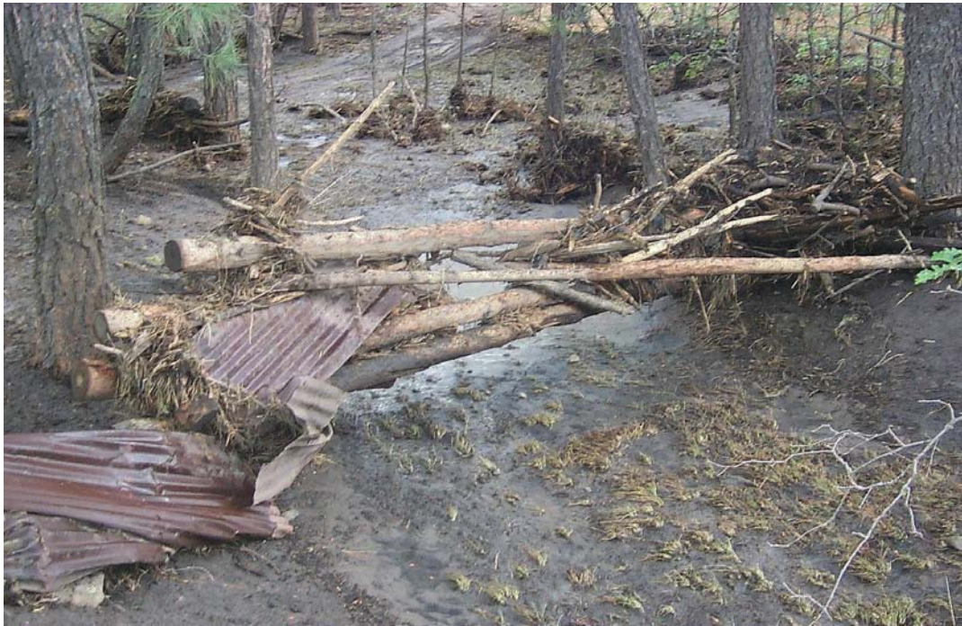
Figure 11.6. The Ice House (post-flood and post-fire).
