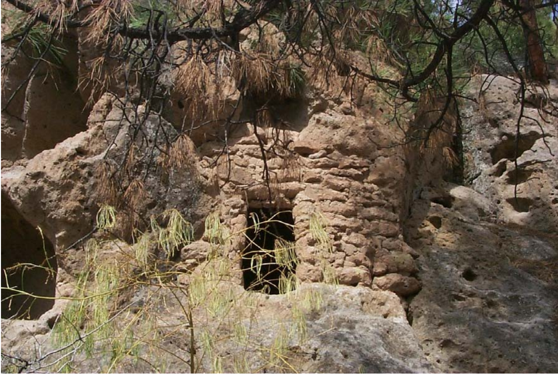
Figure 9.13. LA 16801, a masonry walled cavate with a snag recommended for removal in the foreground.
