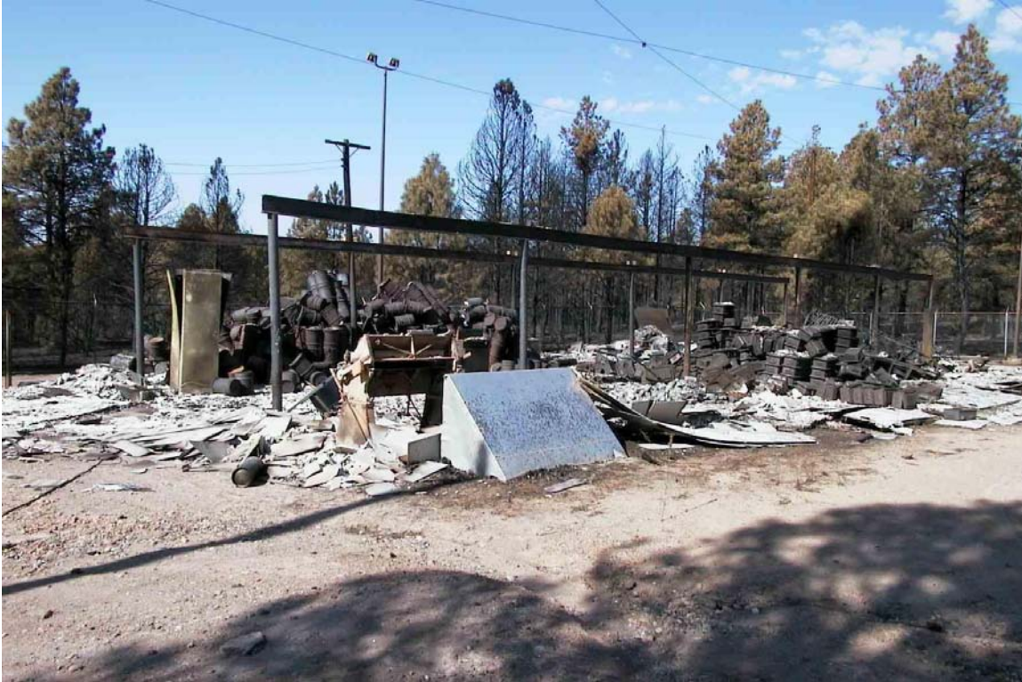
Figure 11.13. TA-40-72 after the Cerro Grande Fire.
