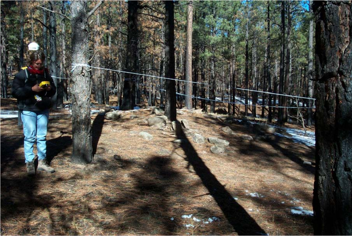
Figure 7.5. LA 86653, J. Nisengard at the two-room structure impacted by the fire.
