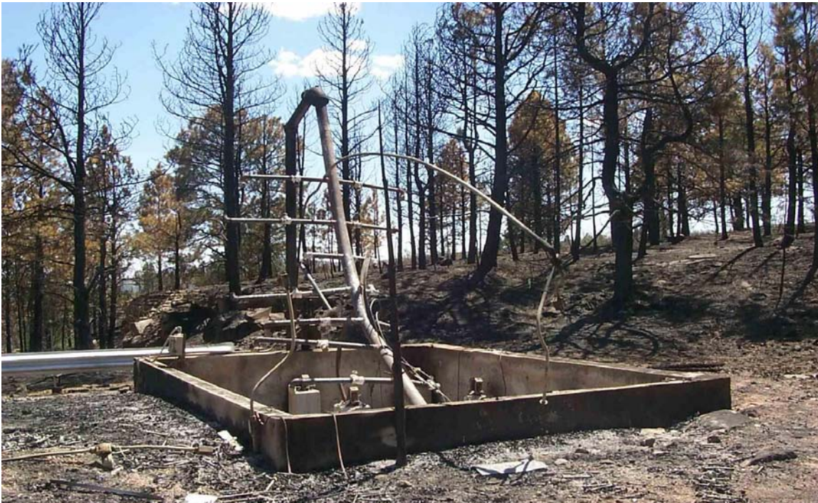
Figure 11.17. TA-16-372 after the Cerro Grande Fire.
