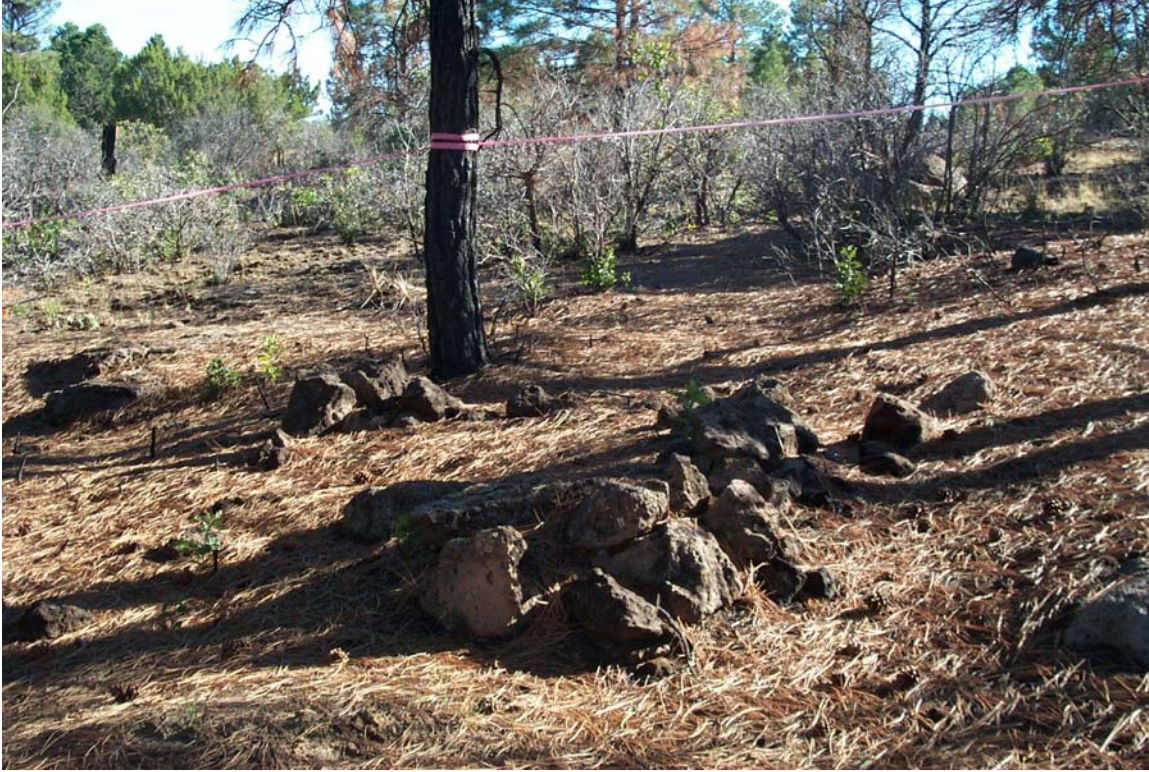
Figure 9.14. LA 16805, a one- to two-room structure impacted by a severe burn, removal of the snag in the background of the photograph is recommended.
