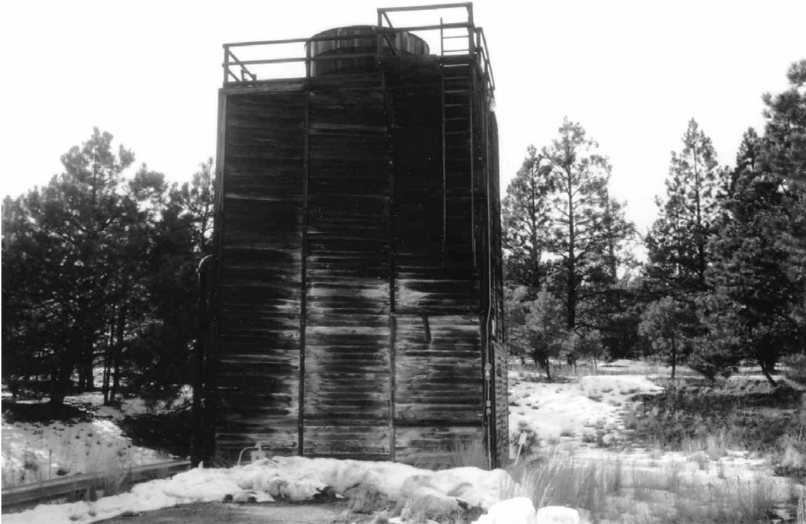
Figure 11.16. TA-16-372 before the Cerro Grande Fire.
