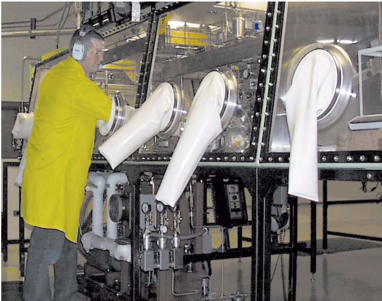
Personnel working at the high-pressure glovebox in WETF.
