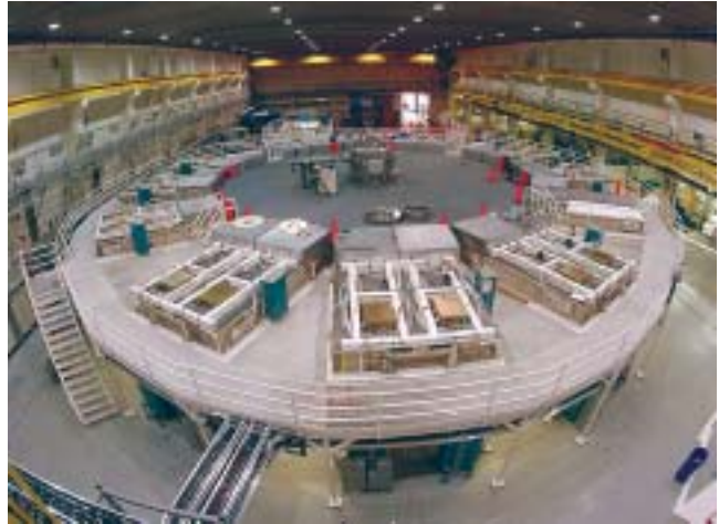
View of the completed Atlas facility.
