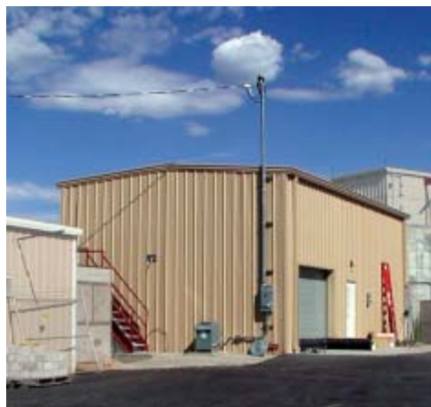
Exterior view of the new ICE House Control Room.
