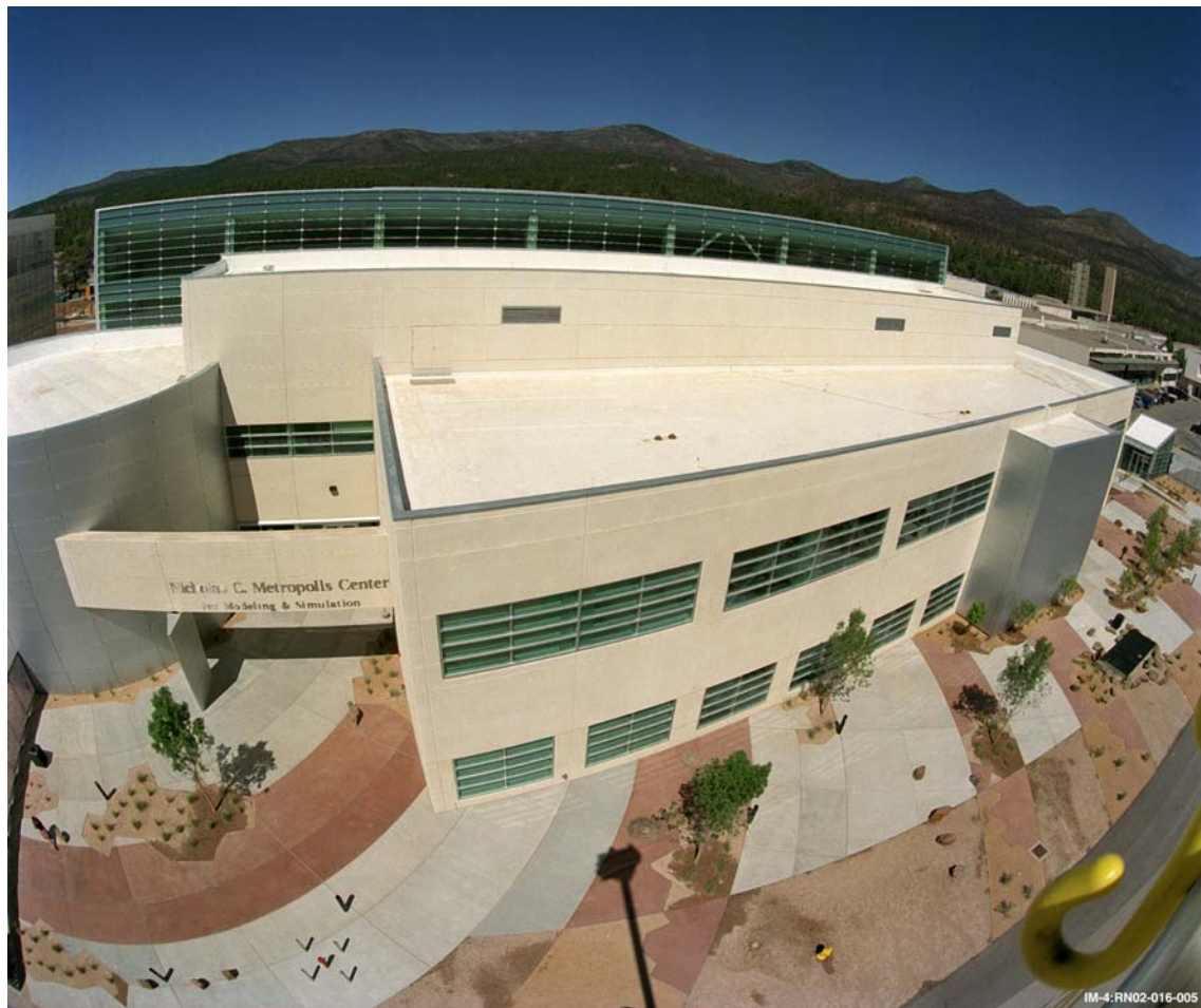
The Nicholas C. Metropolis Center for Modeling and Simulation (Strategic Computing Complex).
