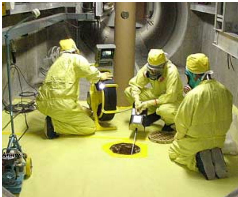
Above: New cooling towers at LANSCE Left: At the Lujan Center, mercury contamination was discovered in the drain system and 1,900 feet of drain was inspected and cleaned
