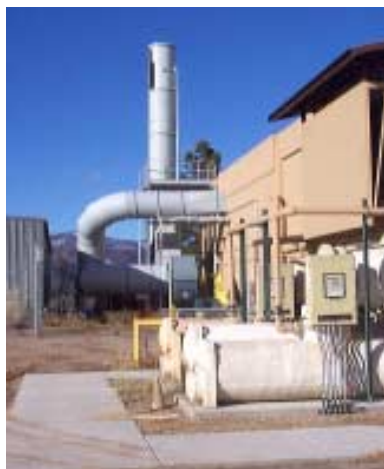
Beryllium collection system at the Sigma Complex
