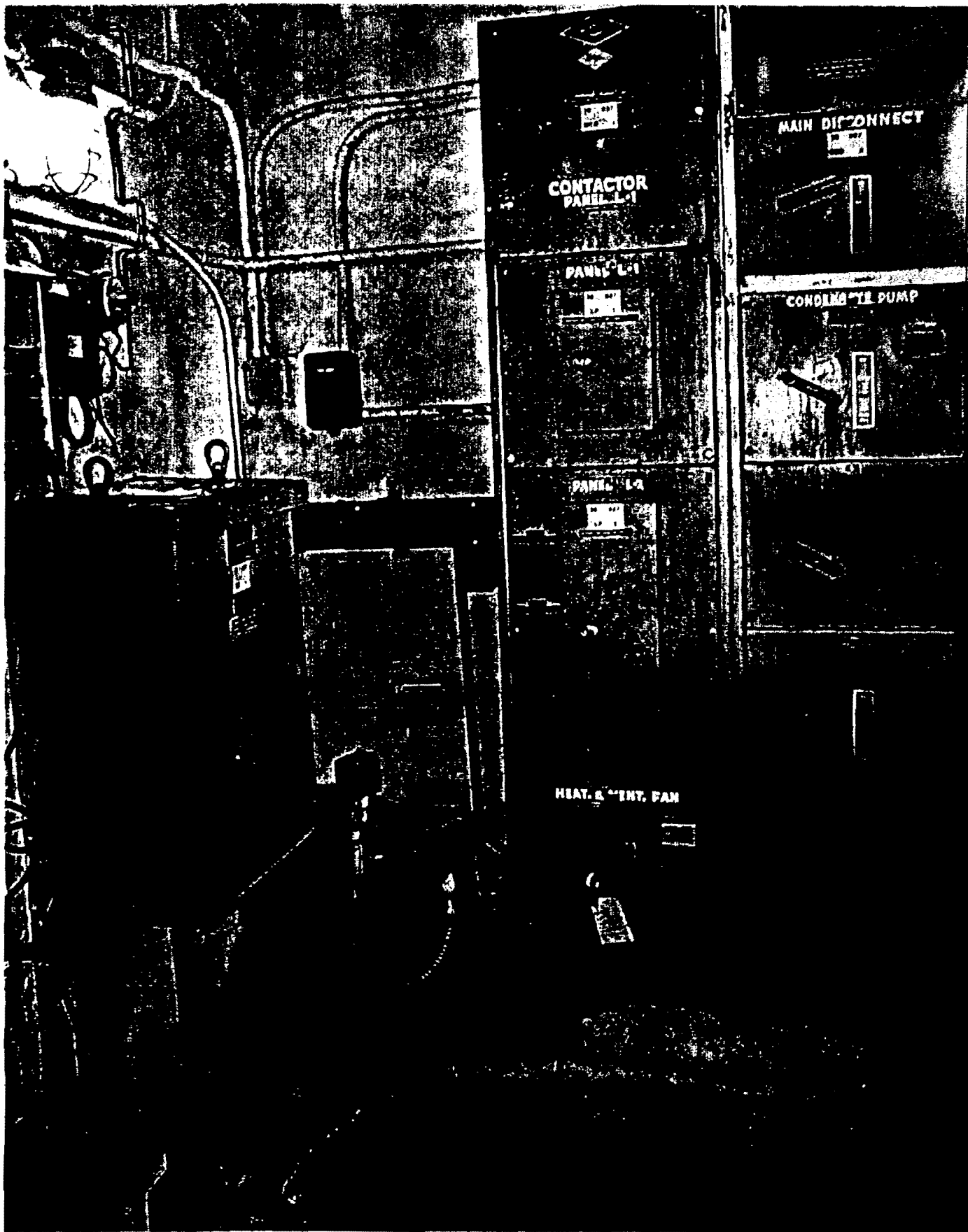
TA-16-437 Utility Room SWMU #16-026(x)
