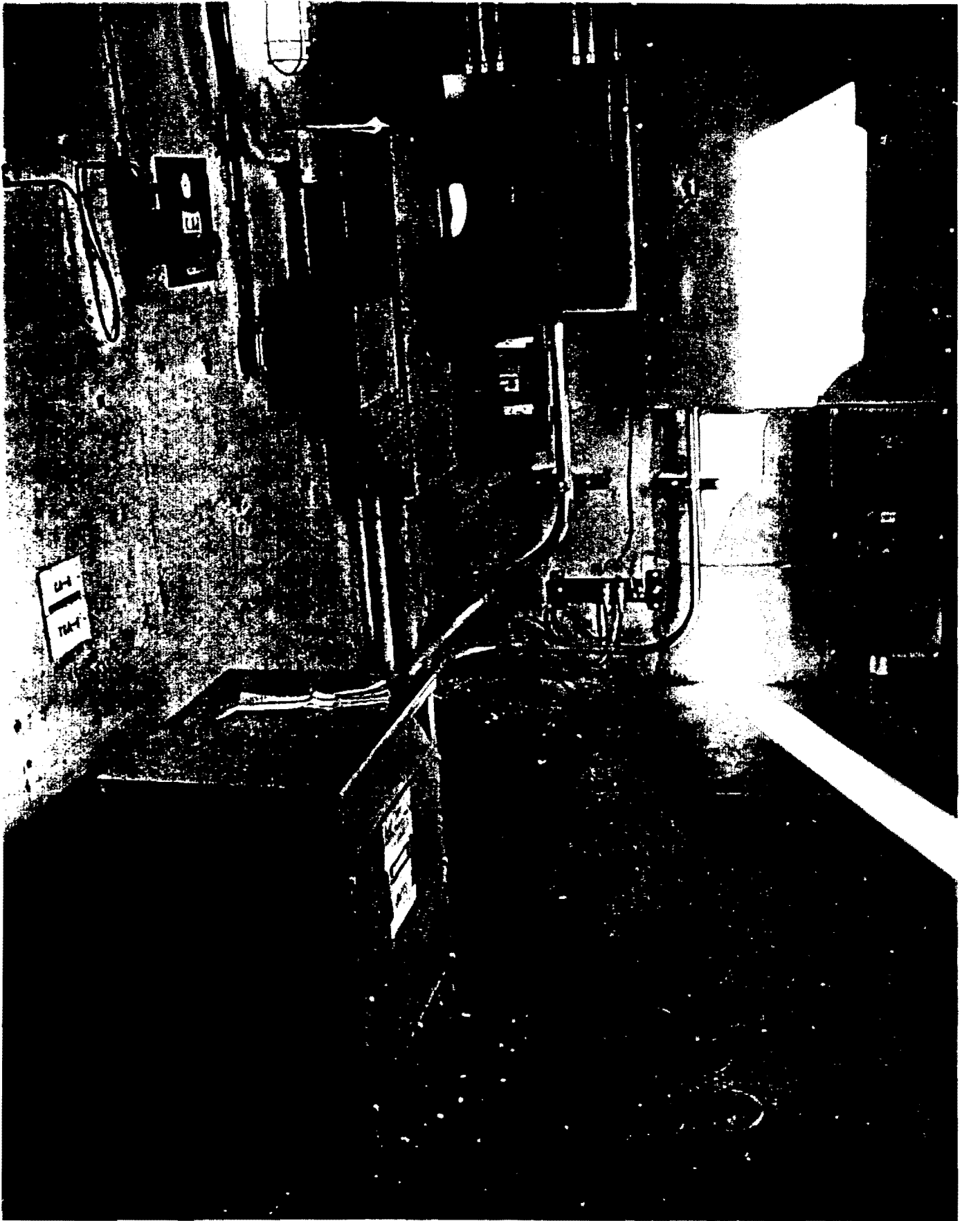
TA-16-415 Utility Room SWMU #16-026(e2)
