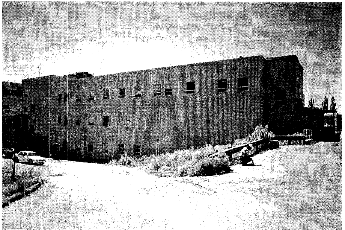
Scyllac Building (TA-3-287) South view
