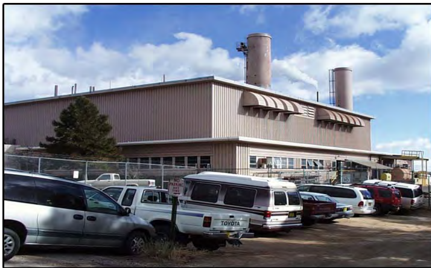
Figure 2.1-1 TA-3 power plant.
