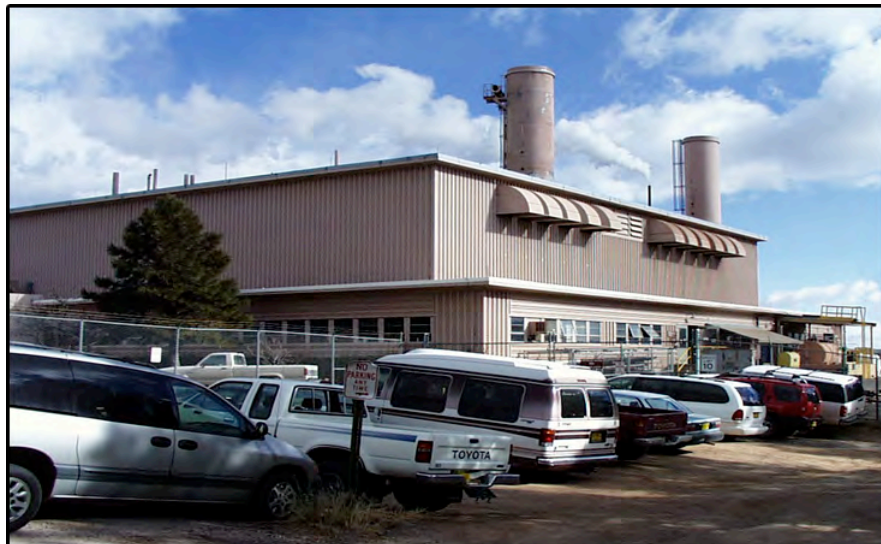
Figure 2.1-1 TA-3 power plant.
