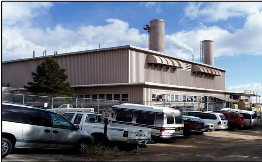
Figure 2.1-1 Main steam plant Technical Area 3 at LANL.
