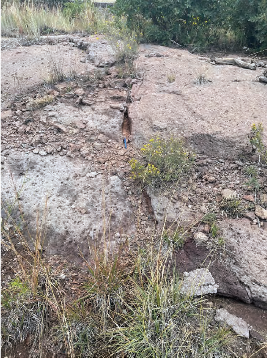
Just south of southern fence at TA-60, Building 17 at road cut, facing north
