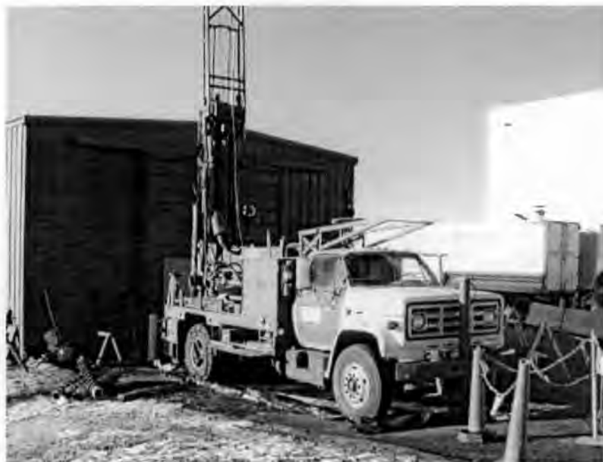
Figure 2.1-1. CME 75 drill rig.
