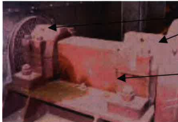
Figure 1. FGR Fan Drive. Remove the shaft guard located in the middle of the drive. The two zerk plugs are located on each of the two bearings.
