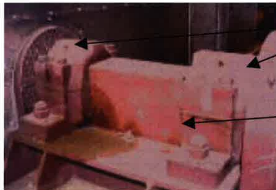
Figure 1. FGR Fan Drive. Remove the shaft guard located in the middle of the drive. The two zerk plugs are located on each of the two bearings.
