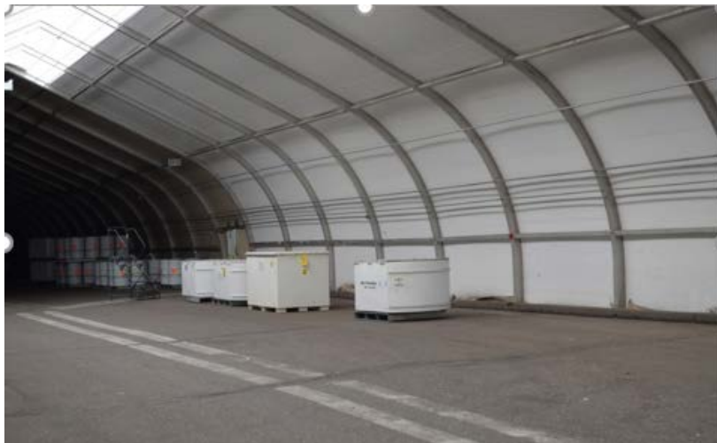
Figure 3-3: Container Storage at Permitted Storage Area
