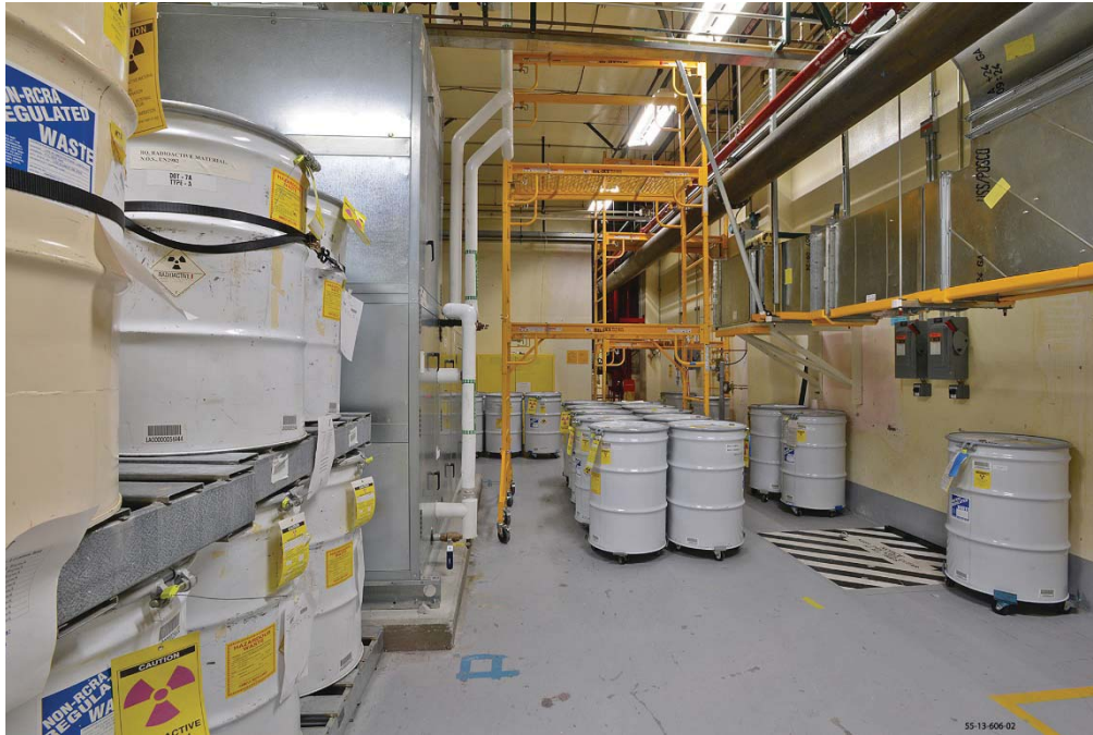
TA-55-4, Basement, Process Code S01, Container Storage Unit (B40) (View is looking southeast)
