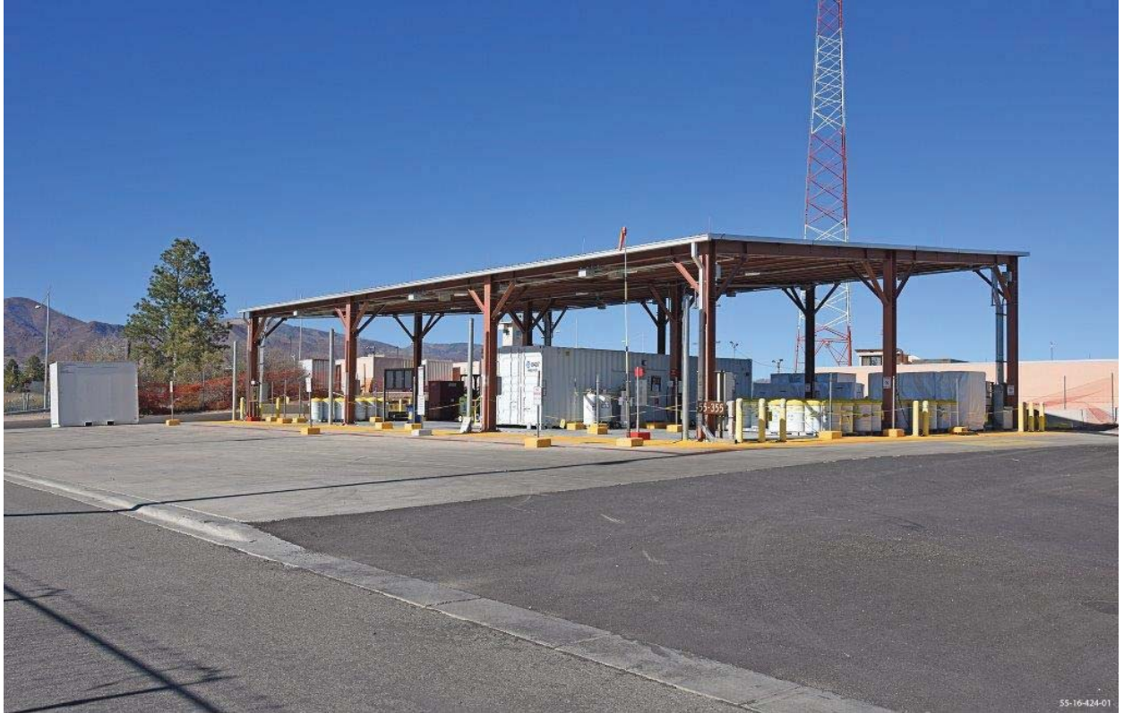
TA-55-0355 Pad Process Code S01, Outdoor Container Storage
