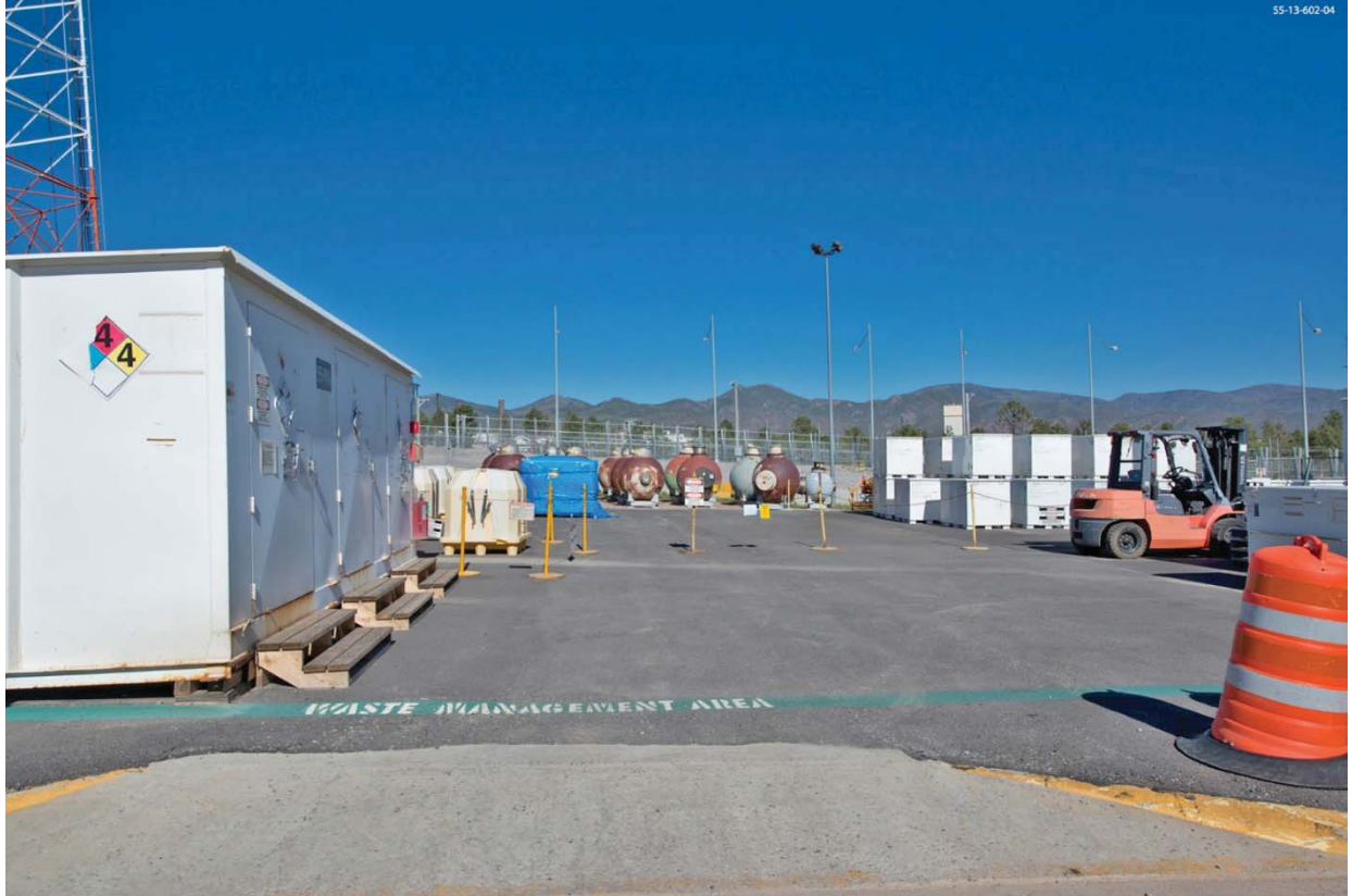
TA-55, Near Building 4, Outdoor Pad, Process Code S01, Container Storage
