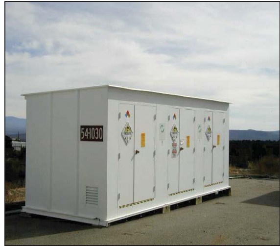
TA-54-1030 Storage Shed Area G, Consolidated Pad No. 5 (Formerly Pad Nos. 5, 7, and 8) Process Code S01, Container Storage
