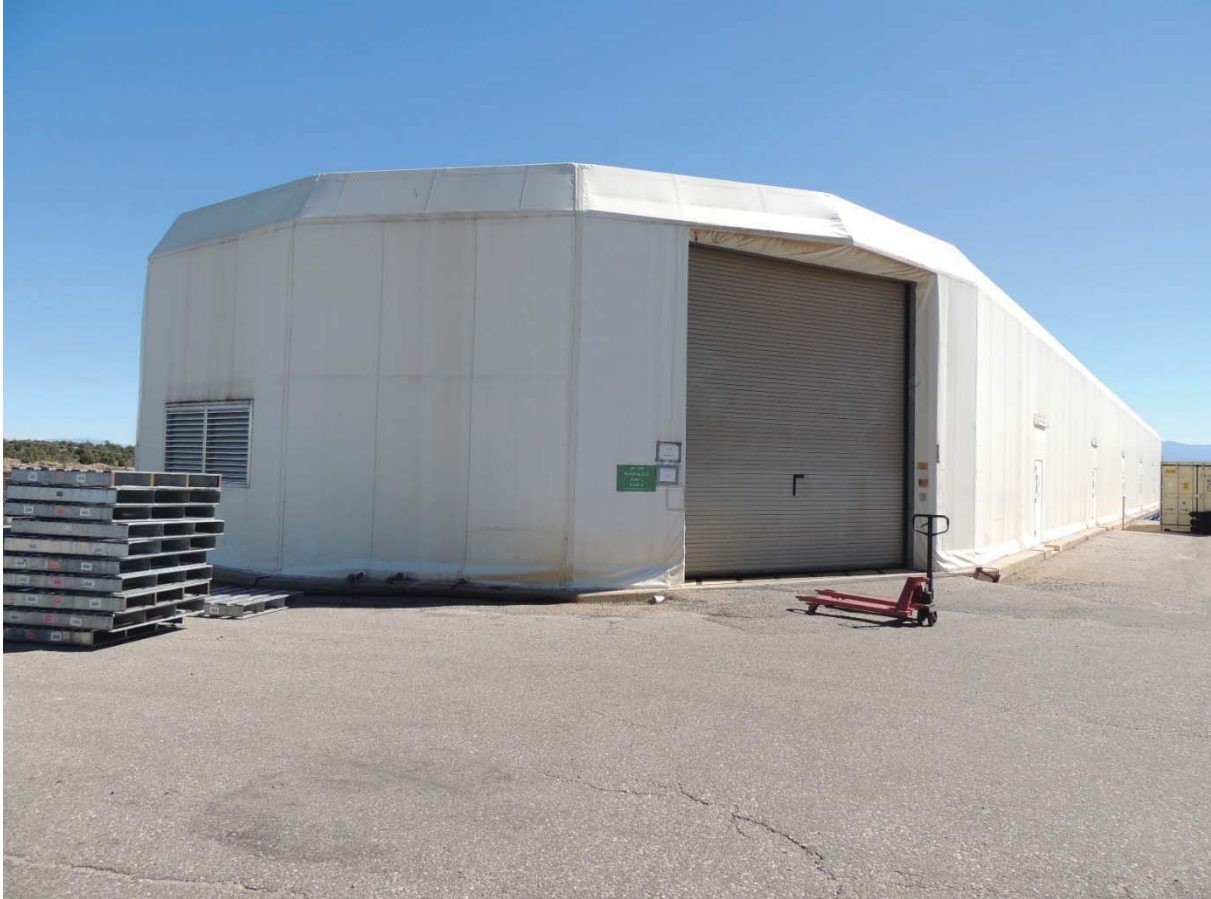
TA-54-215, Area L, Process Code S01, Container Storage Pad/ Storage Dome 215 and Process Code D80, Impoundments B and D
