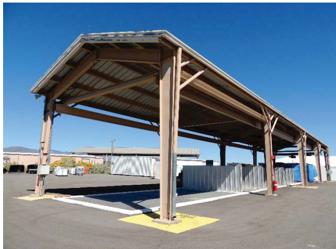
TA-54-32, Area L, Process Code S01, Container Storage Unit (Concrete Containment Structure)
