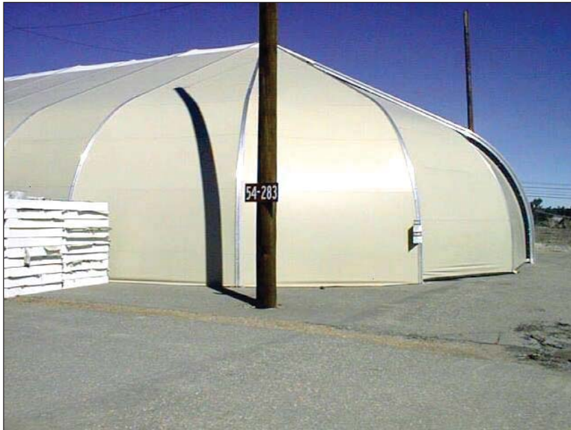
TA-54-283, Area G, Pad No. 6 Storage Dome Process Code S01, Container Storage
