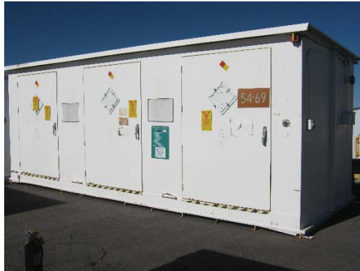
TA-54-69, Area L, Process Code S01, Container Storage (Modular Storage Building 69)
