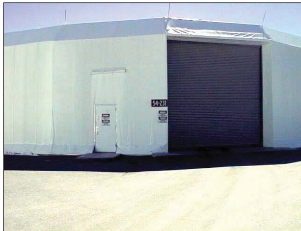
TA-54-231, Area G, Pad No. 9 Storage Dome Process Code S01, Container Storage
