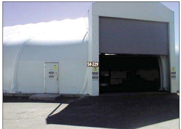
TA-54-229, Area G, Pad No. 9 Storage Dome Process Code S01, Container Storage
