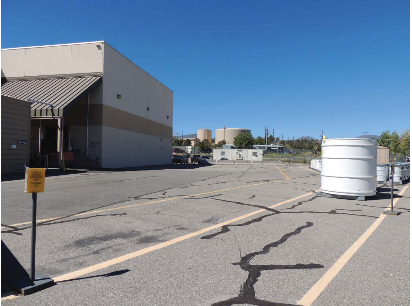
TA-54-38 West Outdoor Pad, Process Code S01, Container Storage Unit
