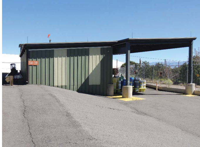
TA-54-39, Area L, Process Code S01, Container Storage Unit
