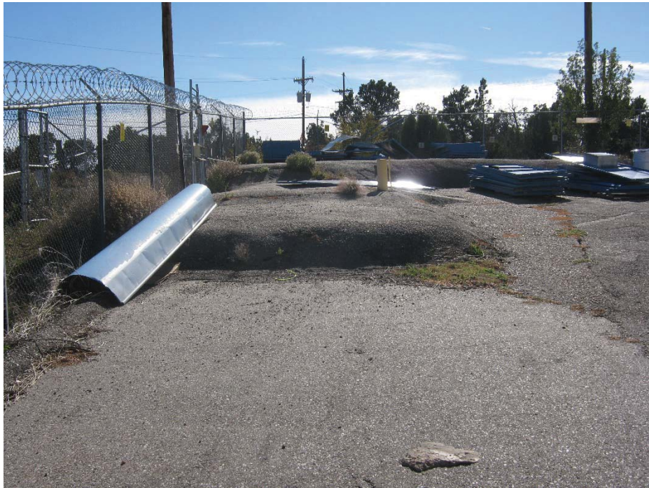
TA-54, Area L, Process Code D80, Disposal Shaft 1 (To be closed)
