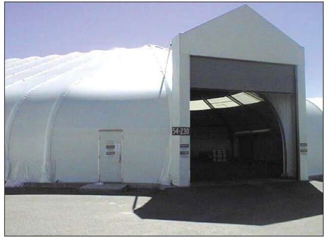
TA-54-230, Area G, Pad No. 9 Storage Dome Process Code S01, Container Storage
