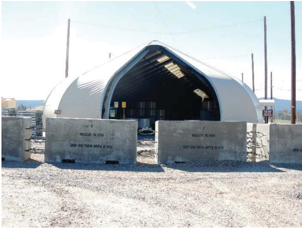
TA-54-49, Storage Dome Area G, Consolidated Pad No. 5 (Formerly Pad Nos. 5, 7, and 8) Process Code S01, Container Storage
