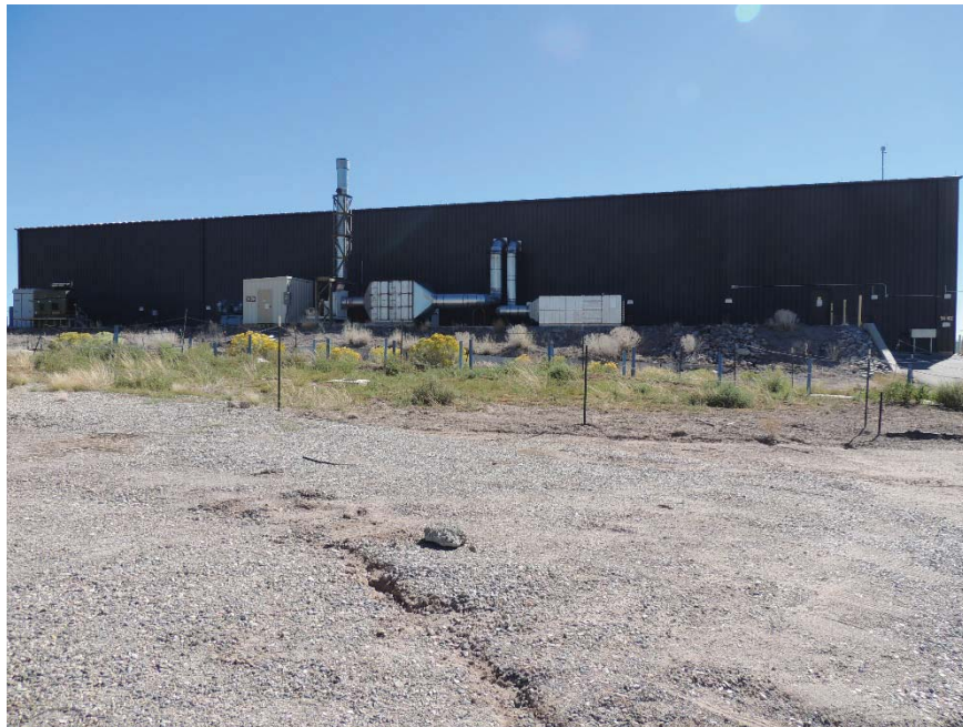
TA-54-412, Area G, Pad No. 1 Decontamination and Volume Reduction System Building Process Code S01, Container Storage
