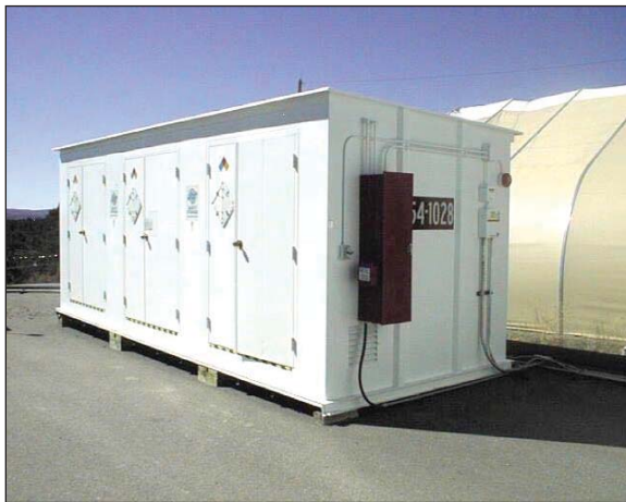
TA-54-1028 Storage Shed Area G, Consolidated Pad No. 5 (Formerly Pad Nos. 5, 7, and 8) Process Code S01, Container Storage
