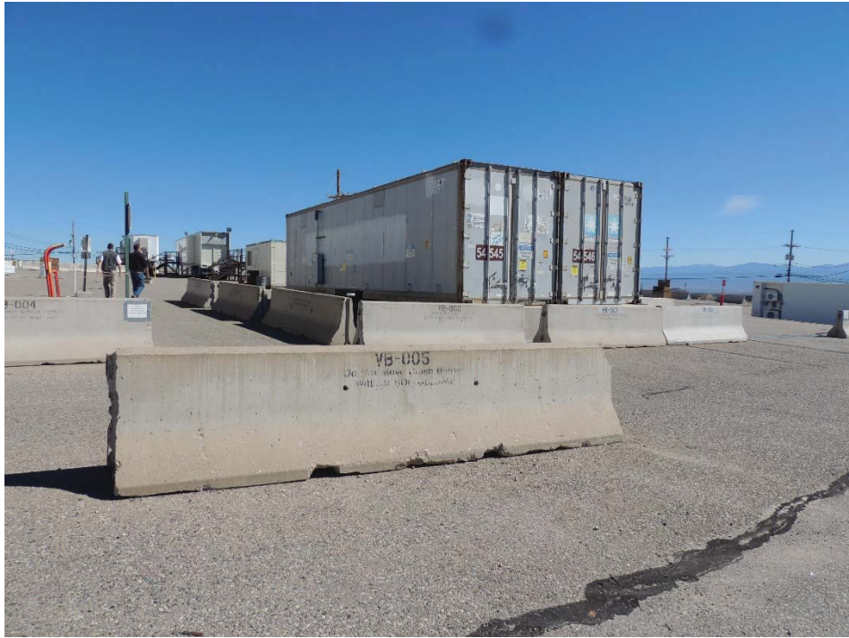
TA-54, Area G, Pad No. 10 Process Code S01, Container Storage
