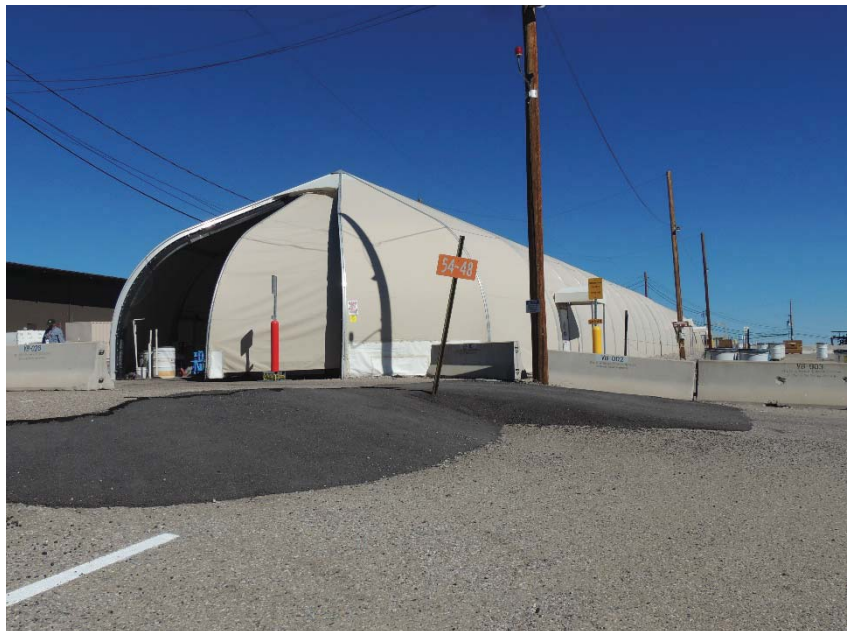
TA-54-48, Area G, Pad No. 3 Storage Dome Process Code S01, Container Storage
