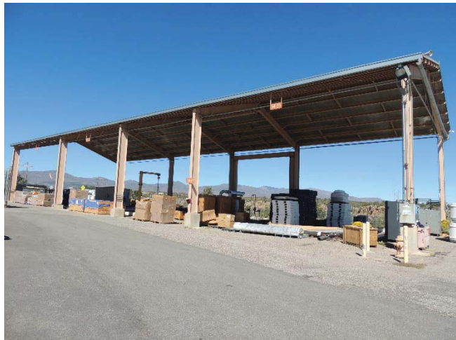
TA-54-35, TA-54-36 and TA-54-58, Area L, Process Code S01, Container Storage Units
