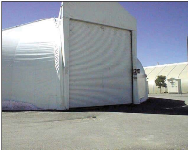
TA-54-224 Storage Dome Area G, Consolidated Pad No. 5 (Formerly Pad Nos. 5, 7, and 8) Process Code S01, Container Storage
