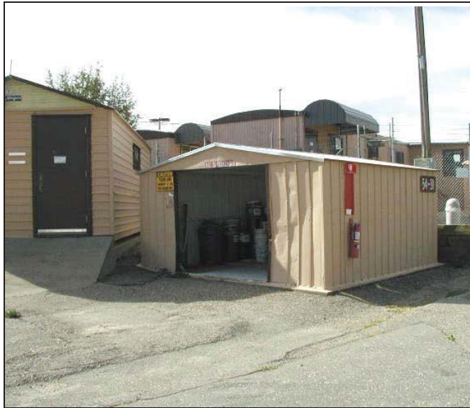
TA-54-31, Area L, Process Code S01, Container Storage Unit
