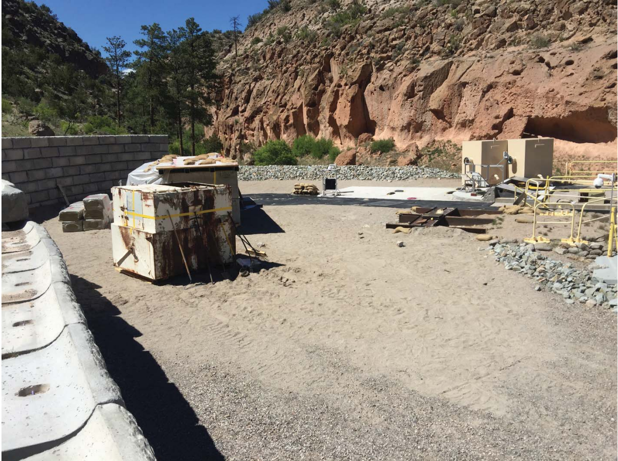
TA-39-6, Process Code X01, Open Detonation Unit (Facing North)
