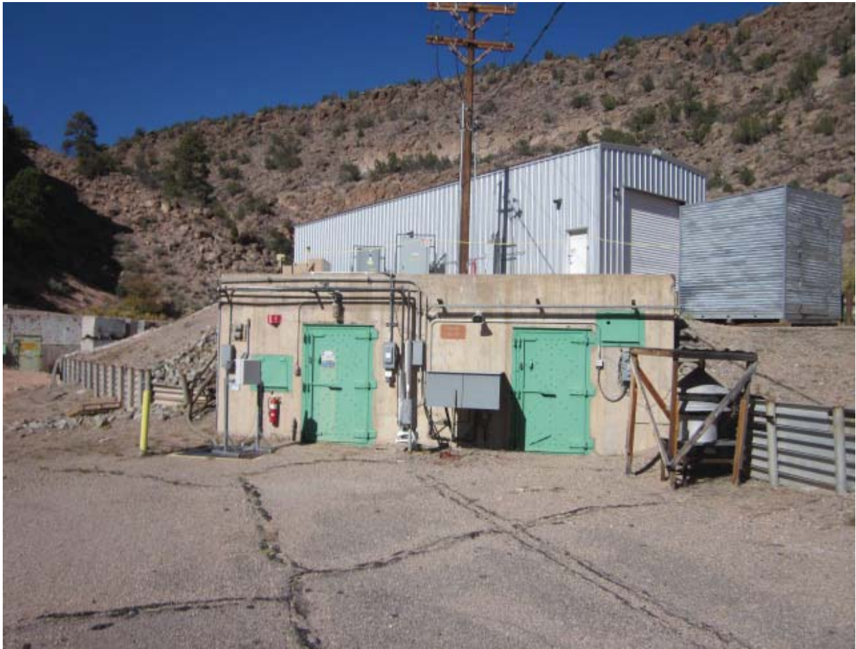
TA-39-57, Process Code X01, Open Detonation Unit
