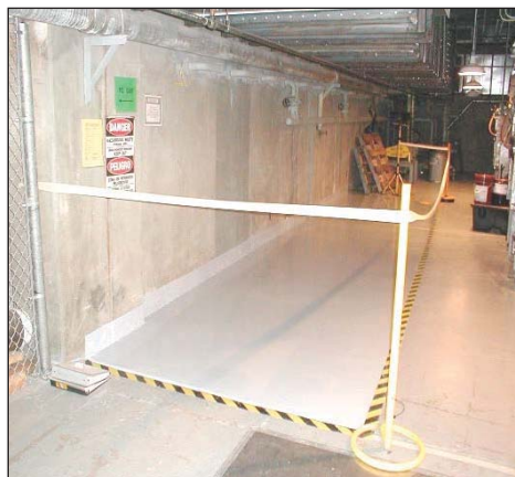
TA-3-29, Wing 9, Basement Room 9030, Process Code S01, Container Storage
