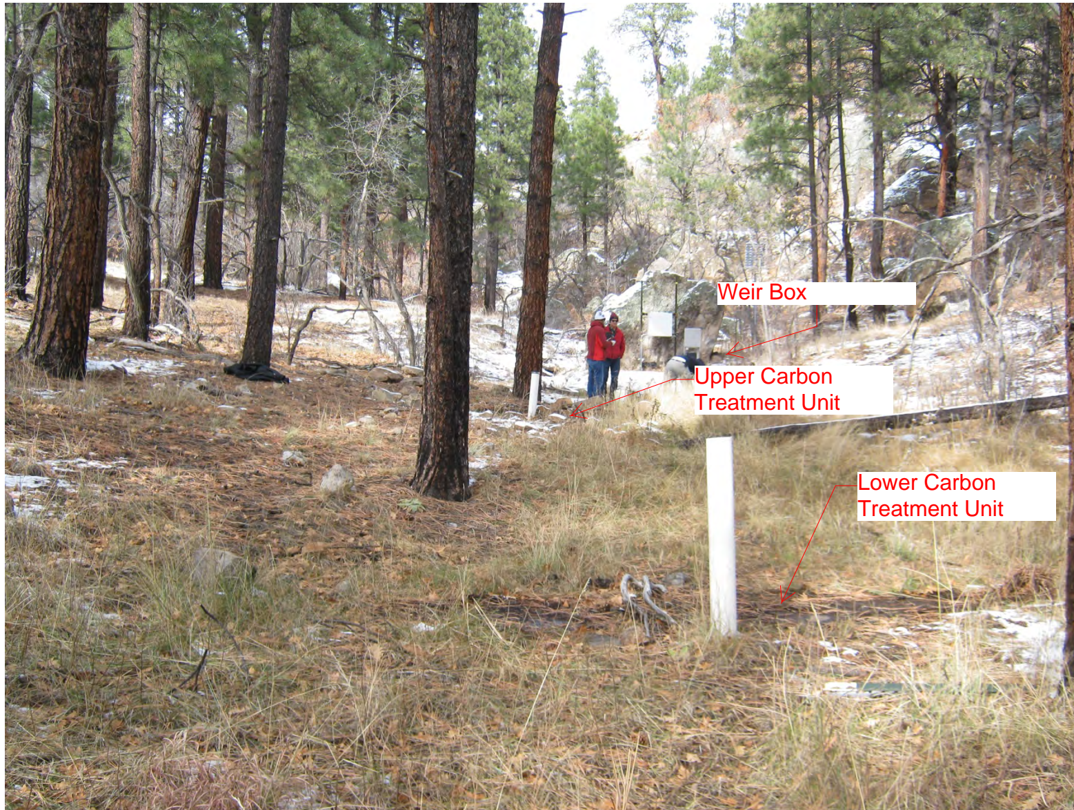
Martin Springs Treatment Units (December 2, 2016)
