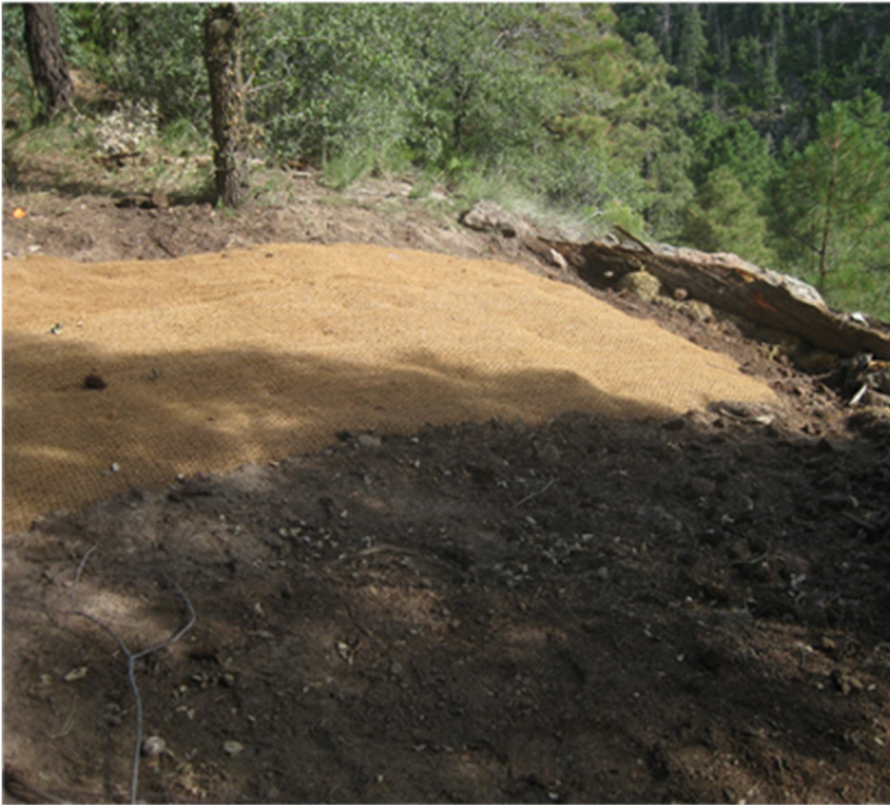
Photo A-5 Post-excavation site restoration within cliff-top area of SWMU 01-001(g)
