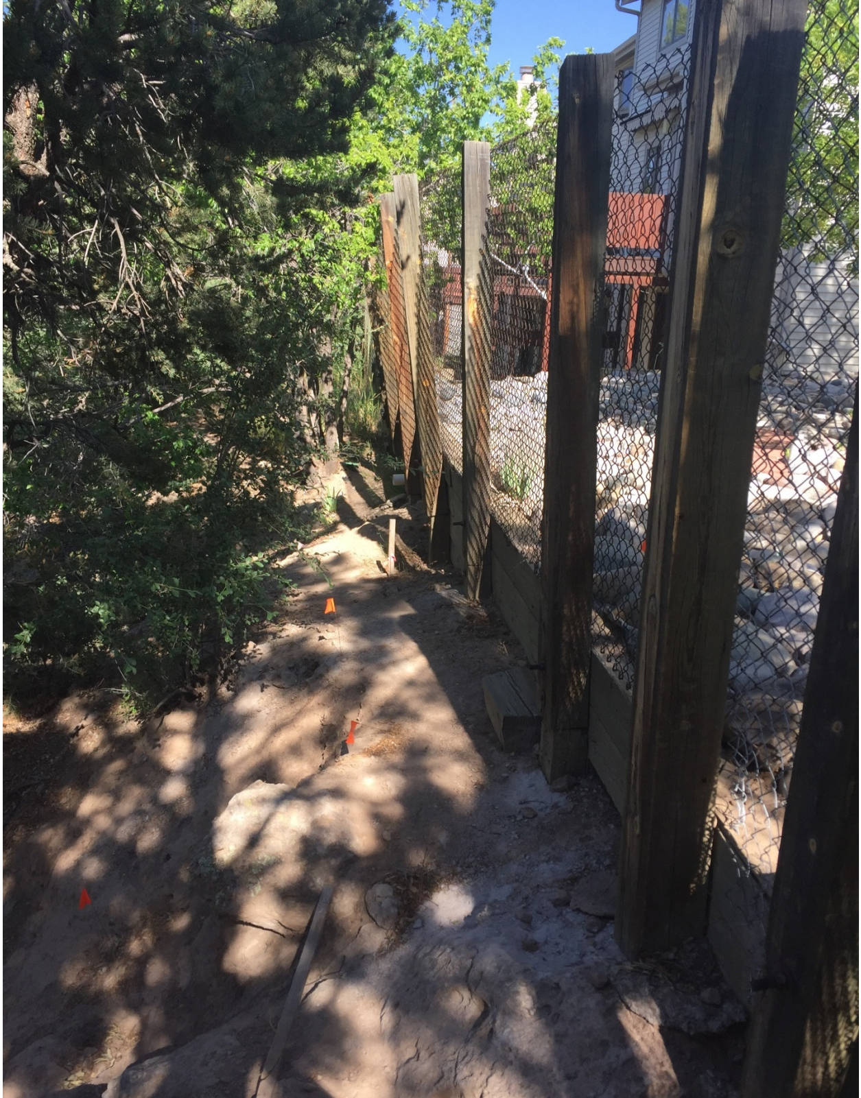
Photo A-6 Area of Concern (AOC) 01-003(b2) site conditions—sampling locations and retaining wall constructed with treated lumber
