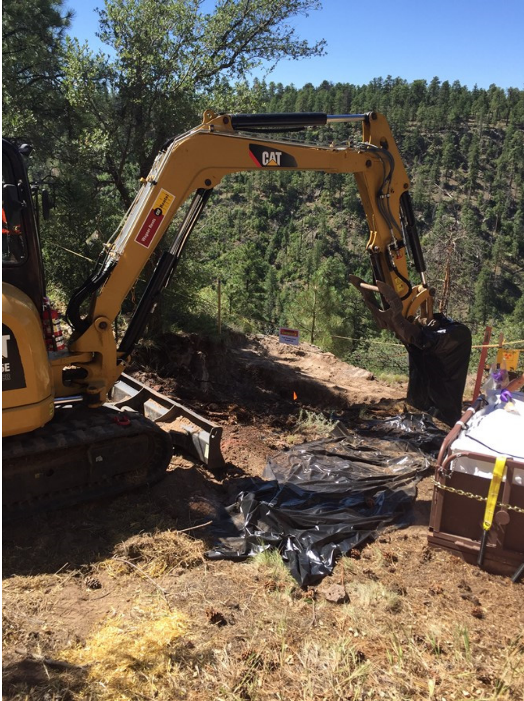
Photo A-2 SWMU 01-001(g) soil excavation
