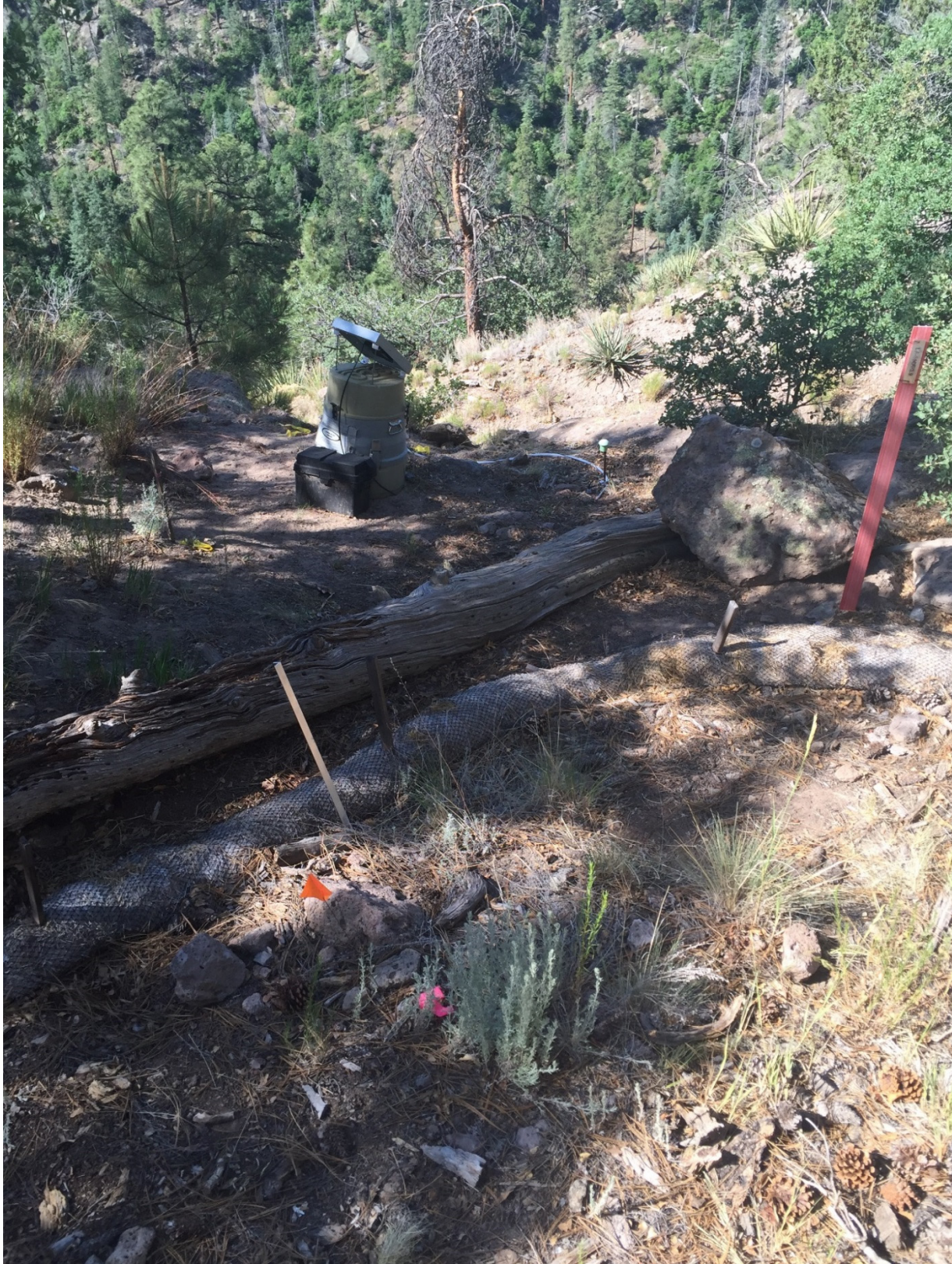
Photo A-1 Solid Waste Management Unit (SWMU) 01-001(g) site conditions (before soil excavation)
