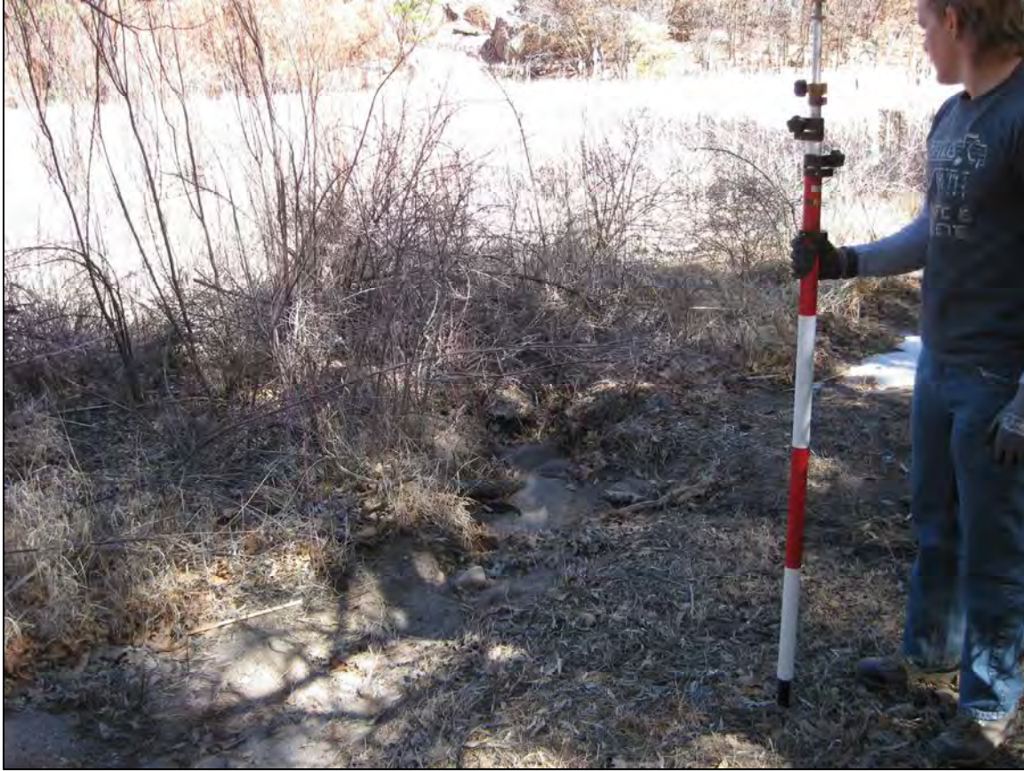
Photo B1-1 Maximum detected negative change (erosion) in reach S-2. March 2017 photo looking to north of the channel incision of 0.7 ft into alluvial fan on southern edge of the reach.
