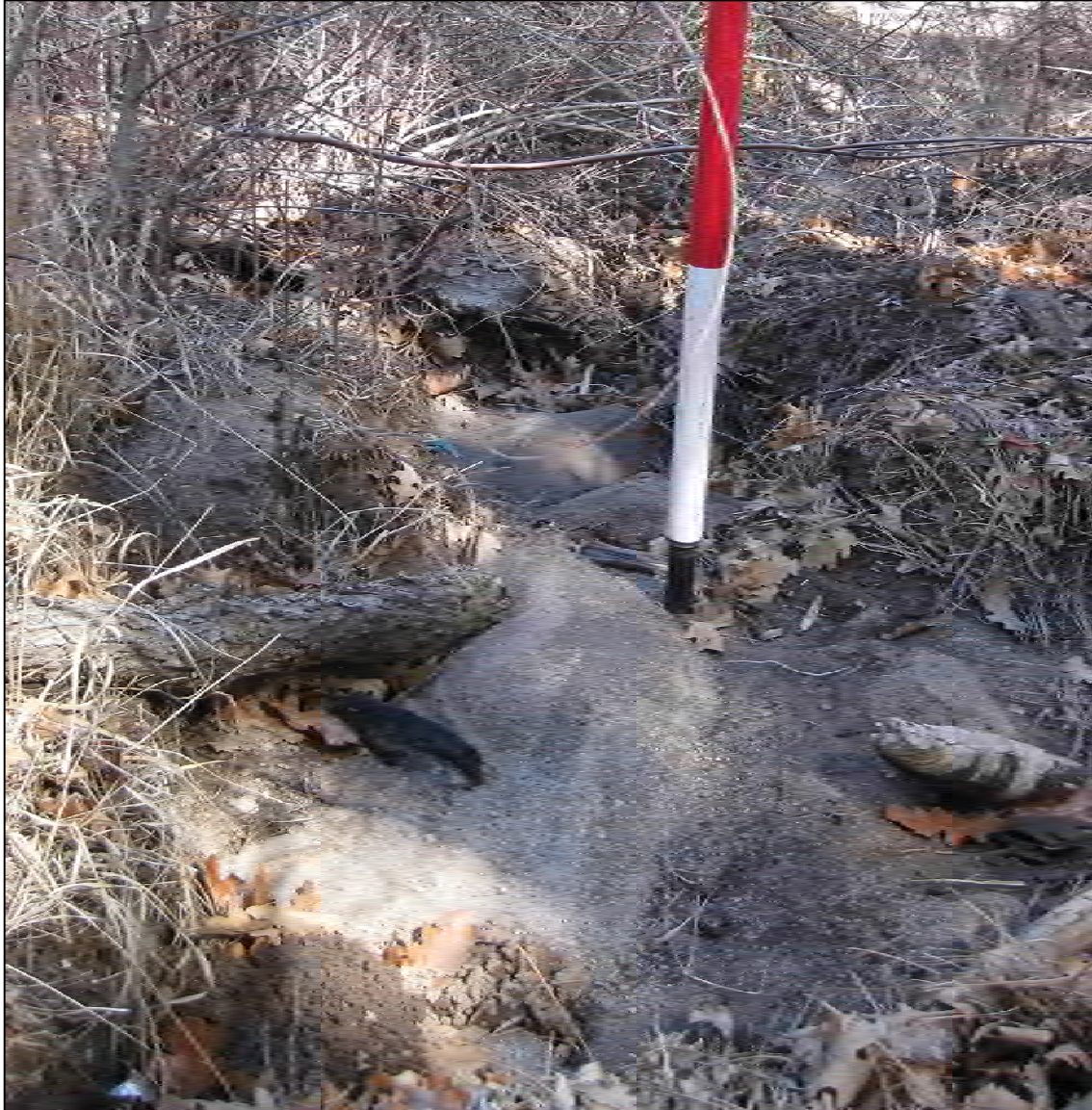
Photo B1-2 Closeup of incised alluvial fan where maximum erosion was noted. March 2017 photo looking north.
