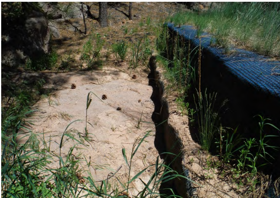
Figure E-2.2-5 June 2016: Upper defense cell, some fine material deposit from Los Alamos County landfill
