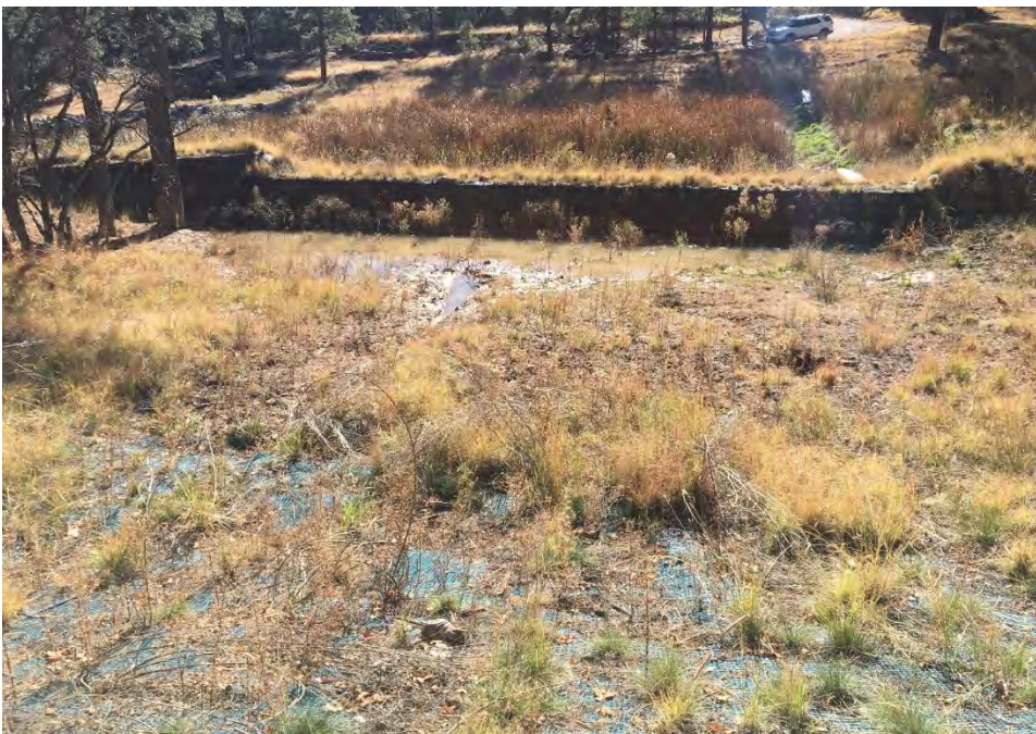
Figure E-2.2-7 November 2016: Lower defense cell operating as designed
