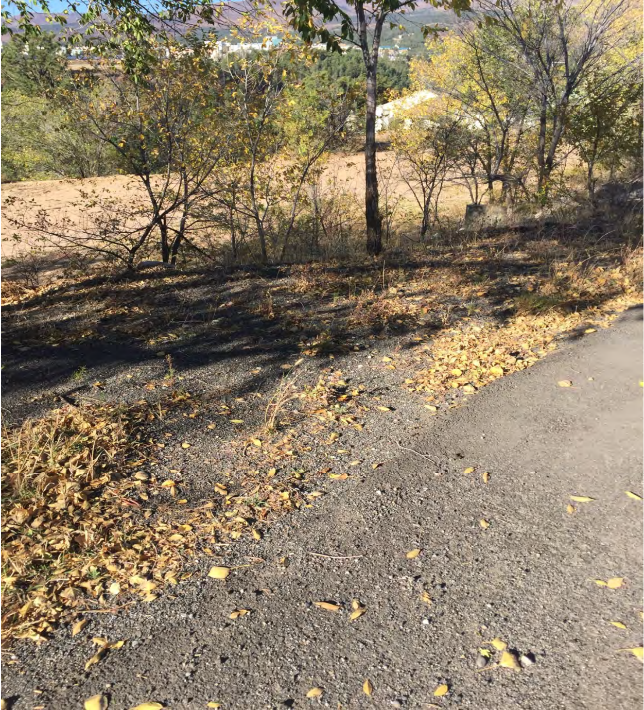
Figure H-5 Asphalt pavement and pieces on the slope of SWMU 01-007(a) above the bench area leading to the canyon slope
