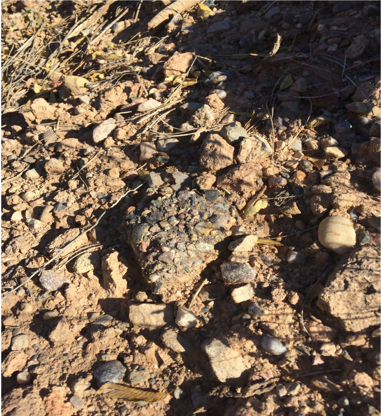
Figure H-3 Pieces of asphalt and debris in the former outfall area of SWMU 01-006(b)
