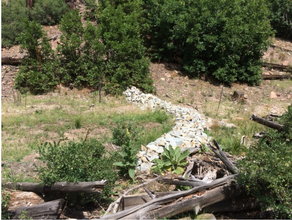
Figure 8 Rock check dam (V00706010025—center of photo) in primary drainage (September 2016). Note established vegetation in channel. Condition of control: excellent.
