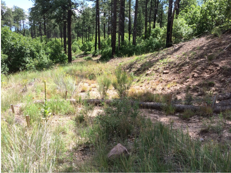
Figure 6 View east of former access road and straw wattle (V007030600028—center of photo) (September 2016). Note established vegetation. Condition of control: very good.
