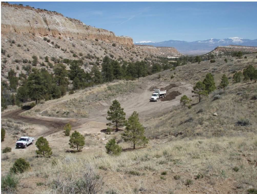
Figure B-9 Emplacement of excavated Los Alamos weir sediments in the borrow pit in 2014
