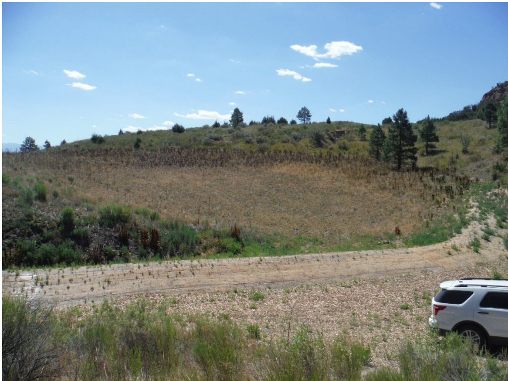
Figure B-13 July 2016 photograph showing current conditions of the sediments placed in the borrow pit
