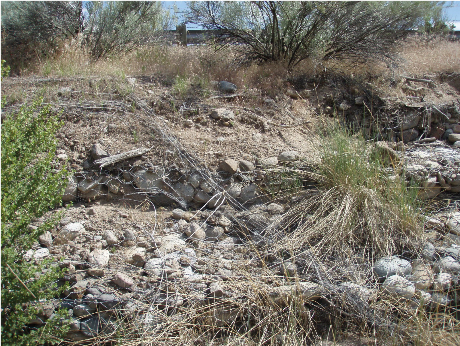
Photo 7 Turf-reinforcing matte present on south side of Los Alamos weir embankment
