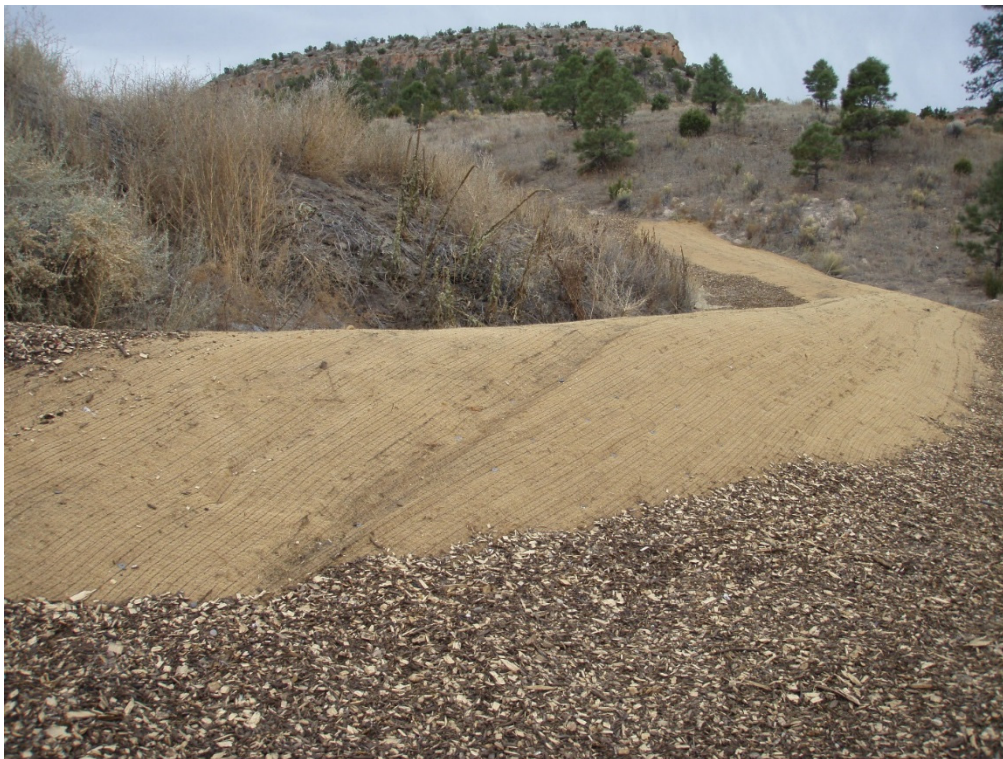
Figure B-11 Runoff retention berm following 2015 maintenance activities
