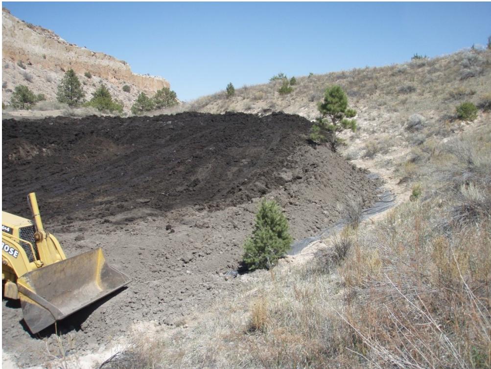
Figure B-7 Emplacement of excavated Los Alamos weir sediments in the borrow pit in 2013
