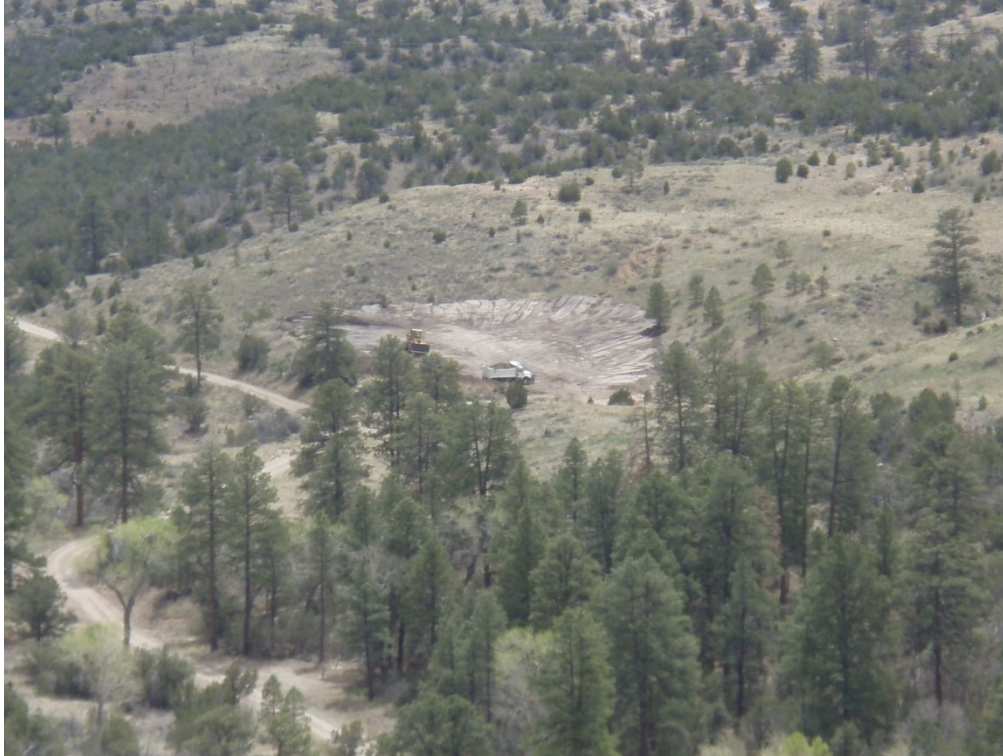
Figure B-10 Emplacement of excavated Los Alamos weir sediments in the borrow pit and contouring of the pit in 2014
