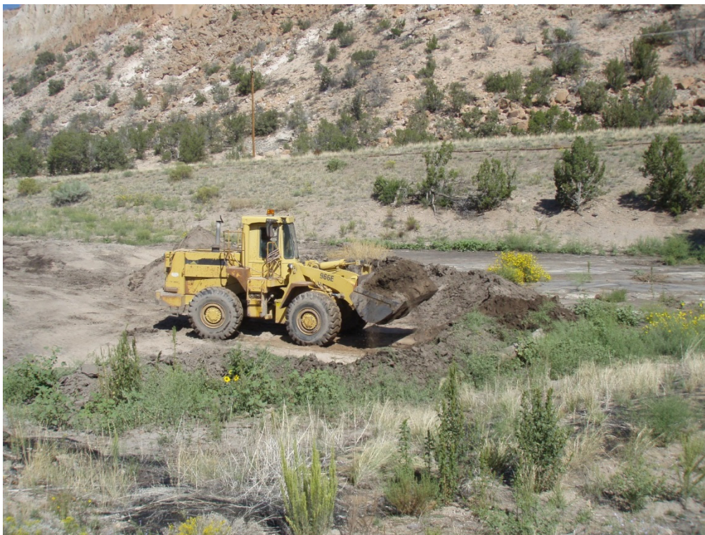
Figure B-2 Excavation of the Los Alamos weir middle basin in 2012
