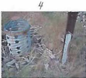
/mc_imageserver/entlan/WO/44555/Standpipe Inlet -image-2016-07-01T19-33-57.2550000Z.jpg
