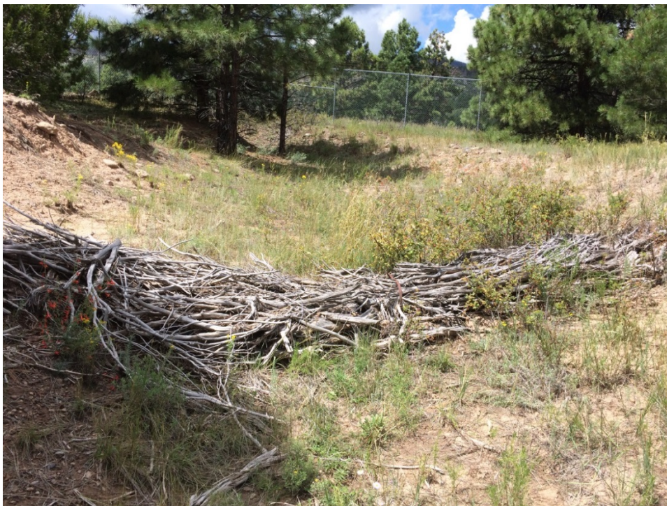
Figure 4 Juniper bale check dam located in drainage channel to 90s Line Pond, September 2016. Note vegetation in channel.
