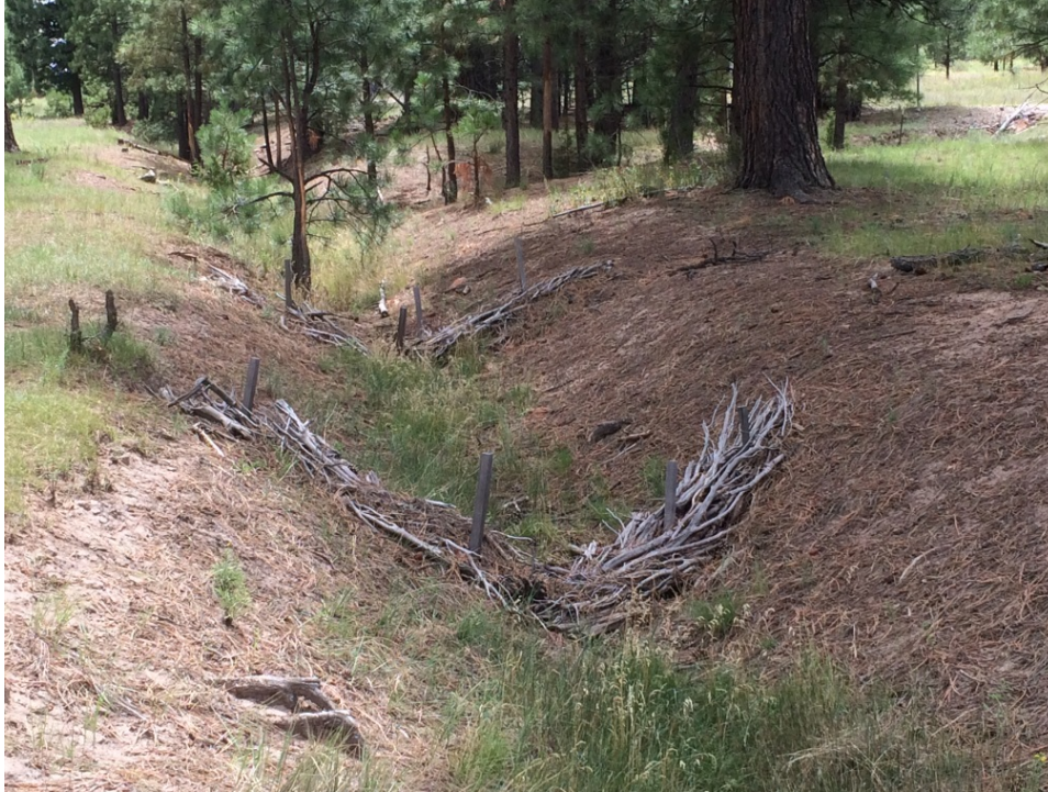
Figure 3 Juniper bale check dams located in drainage channel to 90s Line Pond, September 2016. Note needle cast and vegetation in channel.
