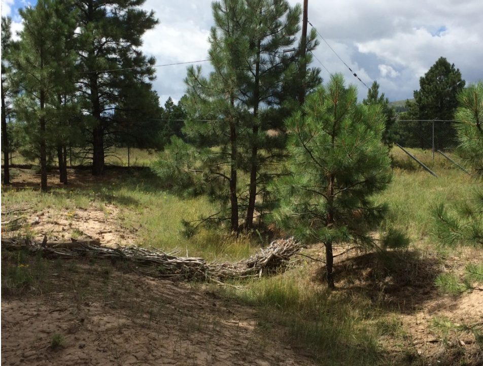
Figure 5 Juniper bale check dam located in drainage channel to 90s Line Pond, September 2016. Note vegetation in channel.
