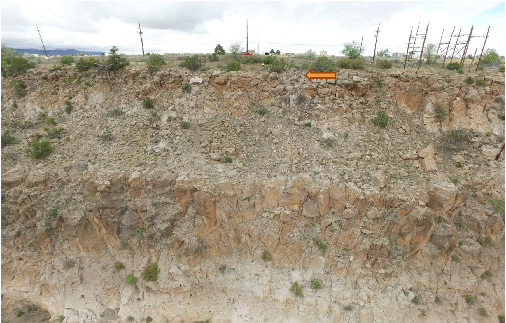
Figure 2 Slope/cliff face at the SWMU 21-022(h) outfall area (arrow)
