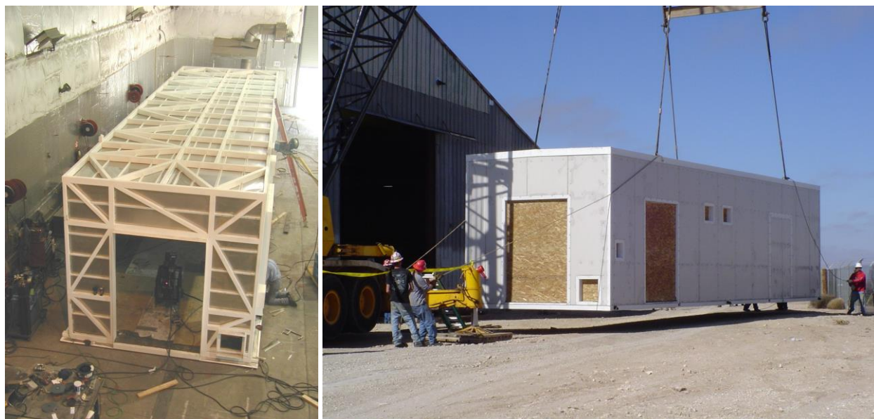
Figure 21 Photos of the nuclear transportainer shell during construction
