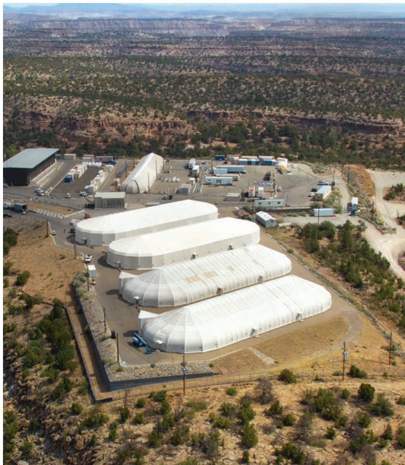
Waste storage domes at Area G
