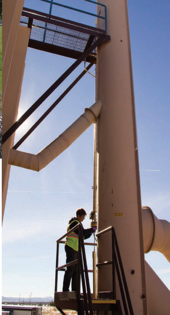
Stack monitoring systems measure airborne emissions of tritium, gases, and particles.
