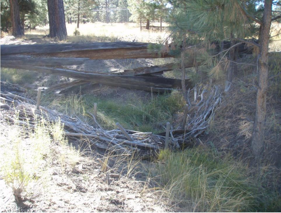
**Figure 5** Juniper bale check dam located in drainage channel to 90s Line Pond, November 2015. Note vegetation in channel.
