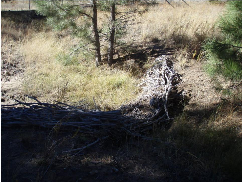
**Figure 4** Juniper bale check dam located in drainage channel to 90s Line Pond, November 2015. Note vegetation in channel.
