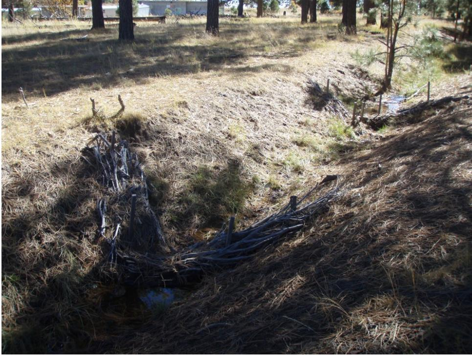
**Figure 3** Juniper bale check dams located in drainage channel to 90s Line Pond, November 2015. Note needle cast and vegetation in channel.
