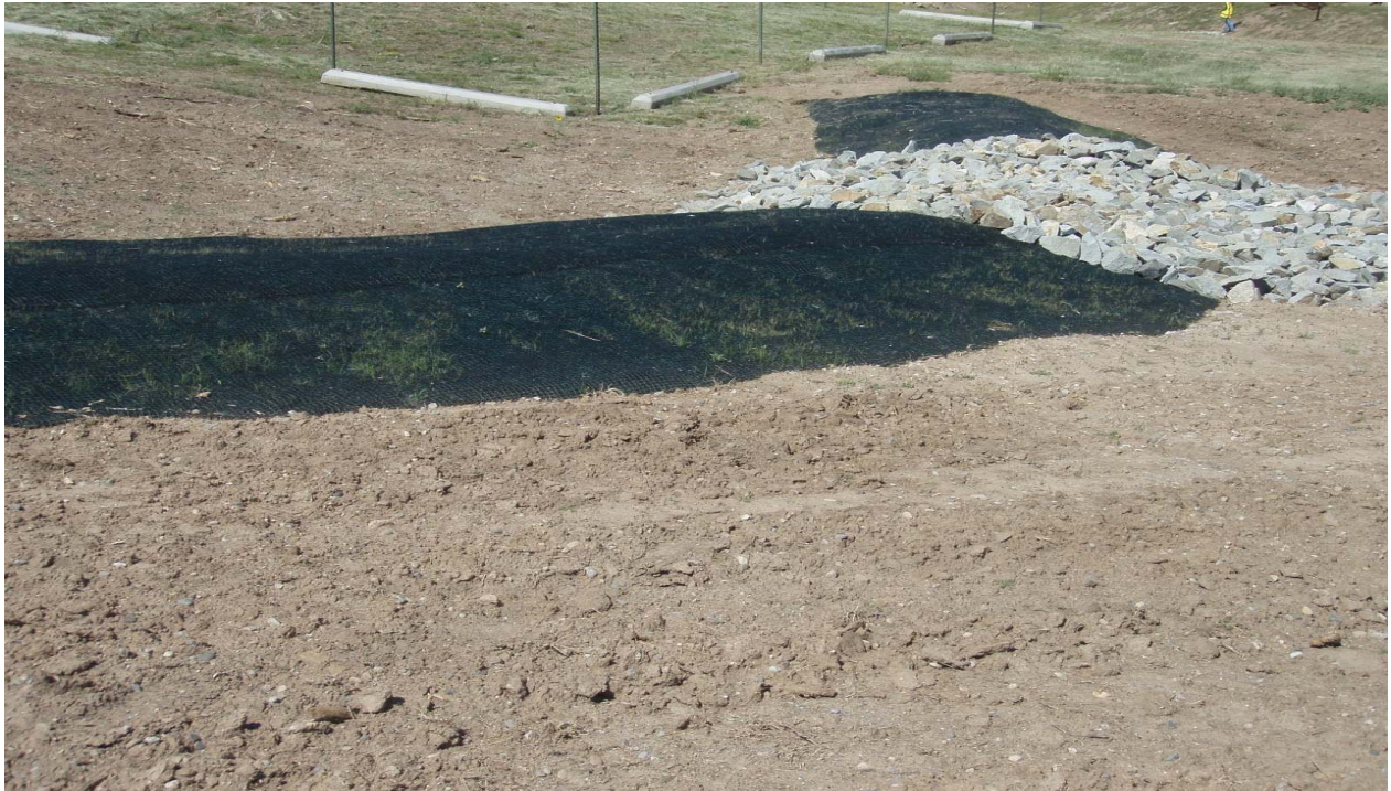
Photo: 49929-14.JPG F00103010026 Berms
