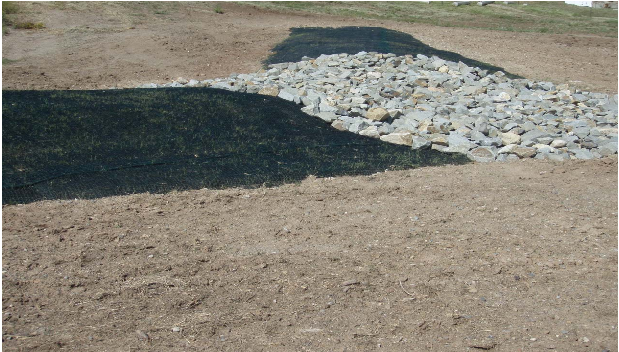
Photo: 49929-13.JPG F00103010025 Berms
