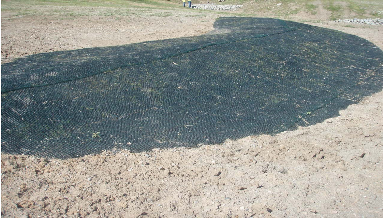
Photo: 49929-15.JPG F00103010027 Berms
