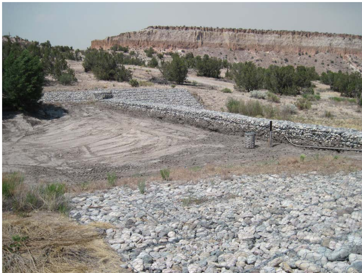
Figure 7-16 LACW structure after sediment excavation in 2014
