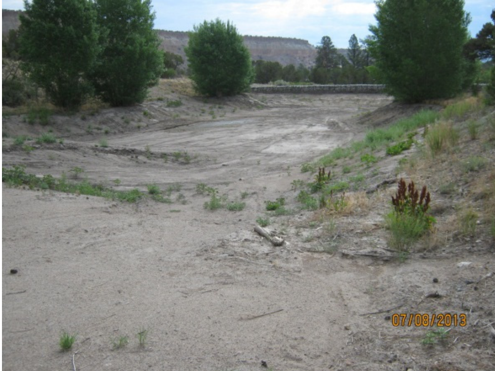
Figure 5 Postexcavation view downcanyon into basin 3
