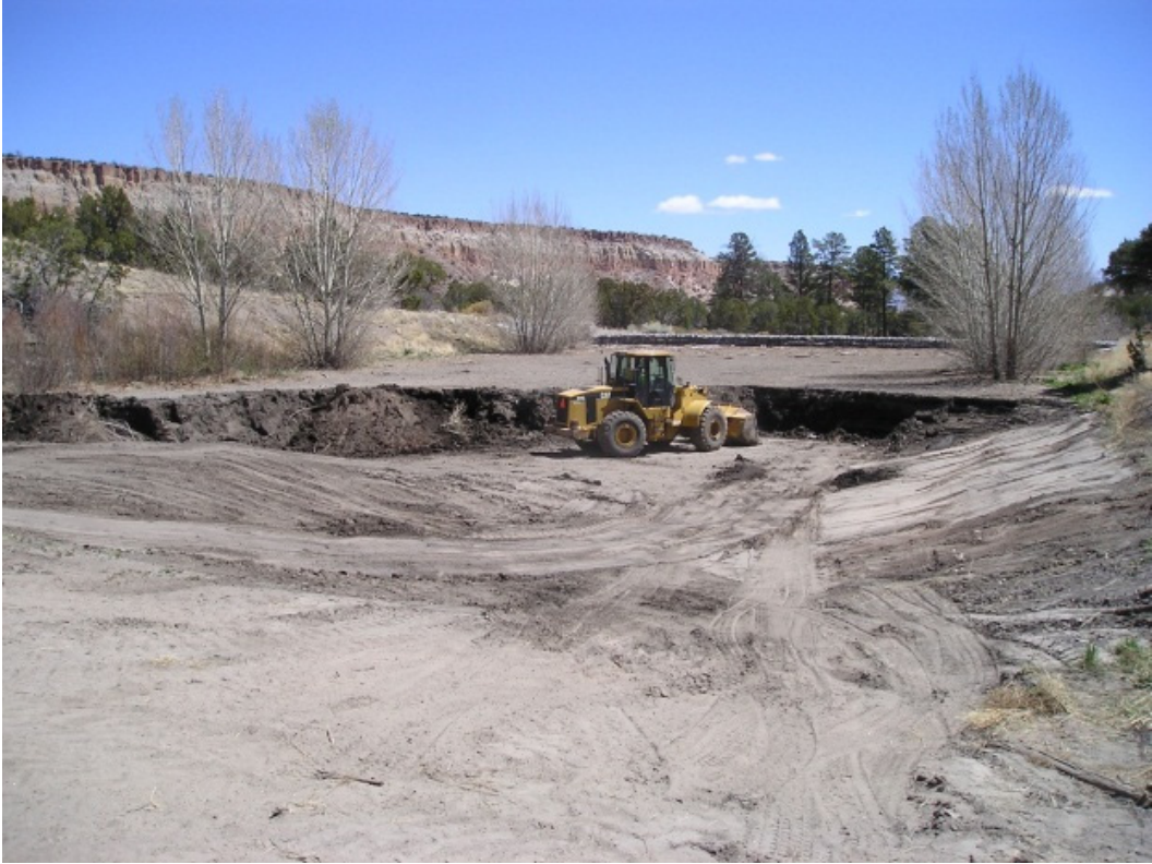
Figure 3 Sediment removal activities in basin 3
