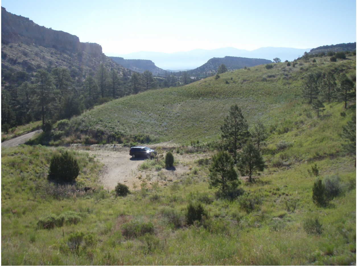
Figure 9 Looking west at sediment placement within the former borrow pit
