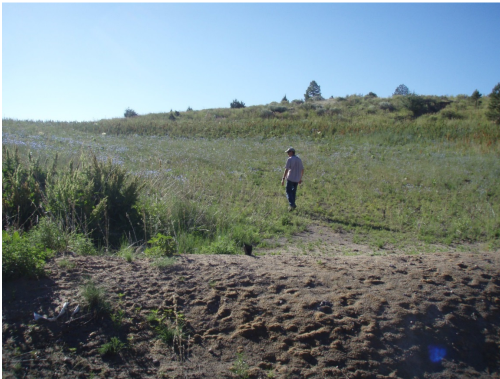
Figure 6 Sediment placement in the borrow pit. Sediment was compacted and contoured to a gradual slope and then hydromulched. Berm is located in foreground of photo.
