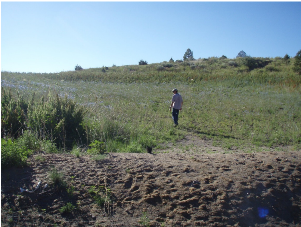
Figure 6 Sediment placement in the borrow pit. Sediment was compacted and contoured to a gradual slope and then hydromulched. Berm is located in foreground of photo.
