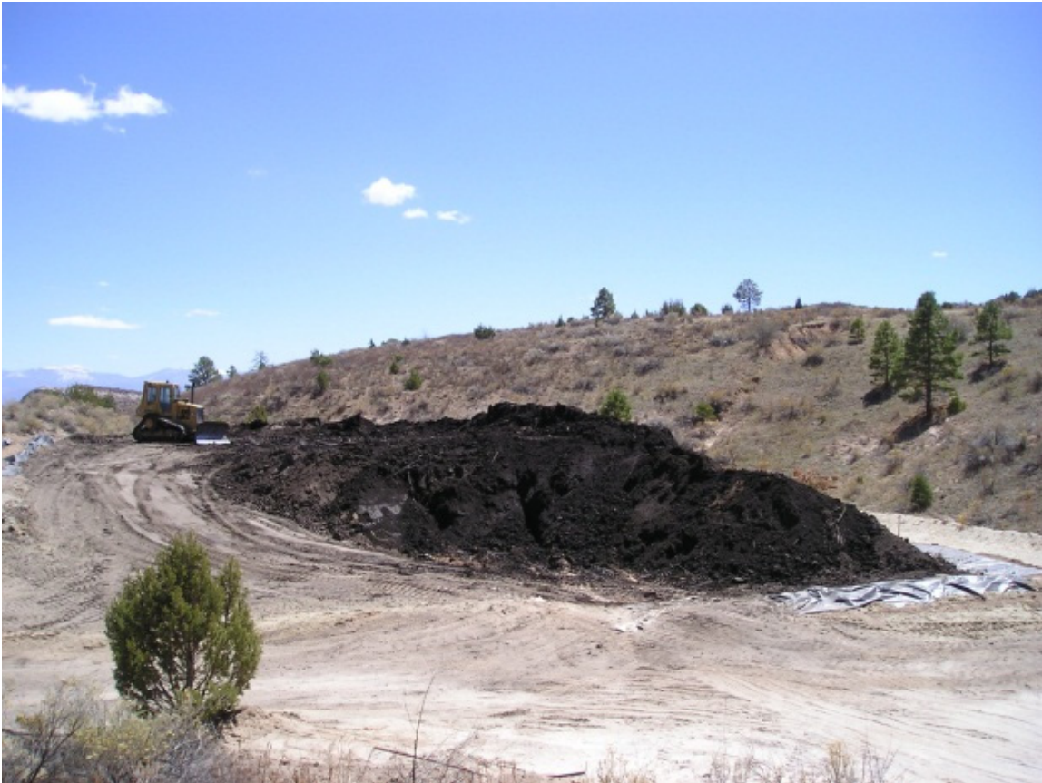
Figure 2 Excavated sediment being placed in former borrow pit in Los Alamos Canyon
