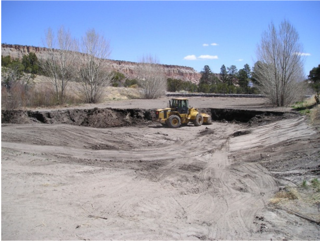
Figure 3 Sediment removal activities in basin 3
