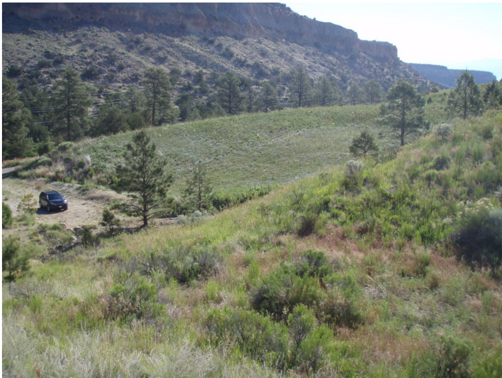
Figure 8 Looking northeast at sediment placement within the former borrow pit. Run-off berm is located at base of slope, just right of vehicle.
