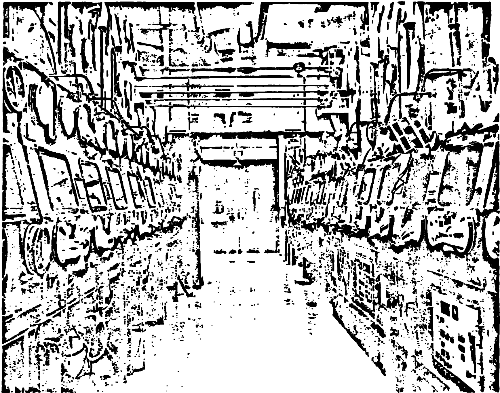
Figure 10. Typical Glovebox Line in Plutonium Facility
