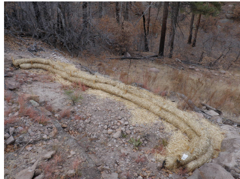
Figure 3 2014 Installation – Straw wattle (V00703060028) on the slope into Fishladder Canyon (11/14/2014)
