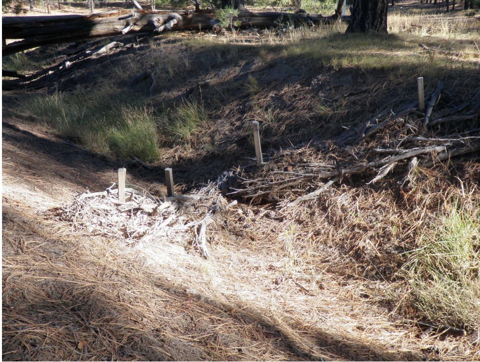
Figure 1 Juniper bale check dam in channel draining to 90s Line Pond, October 2014. Note needle cast and vegetation in channel.
