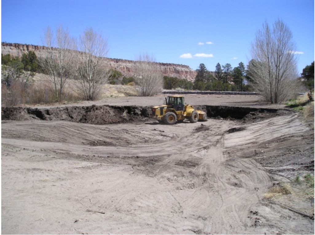
Figure 3 Sediment removal activities in basin 3
