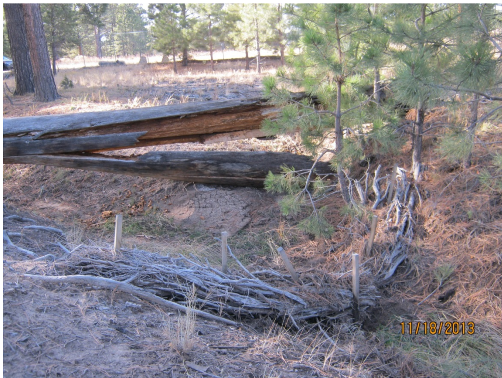
Figure 2 Juniper bale check dam in channel draining to 90s Line Pond, November 2013
