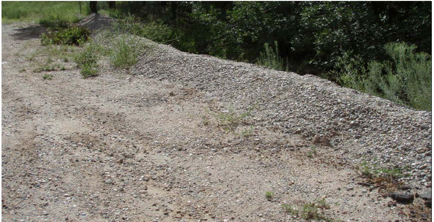
Photo 7600-1.JPG (taken 08/03/10) S00303020008 : Berms - Base Course Berm.
