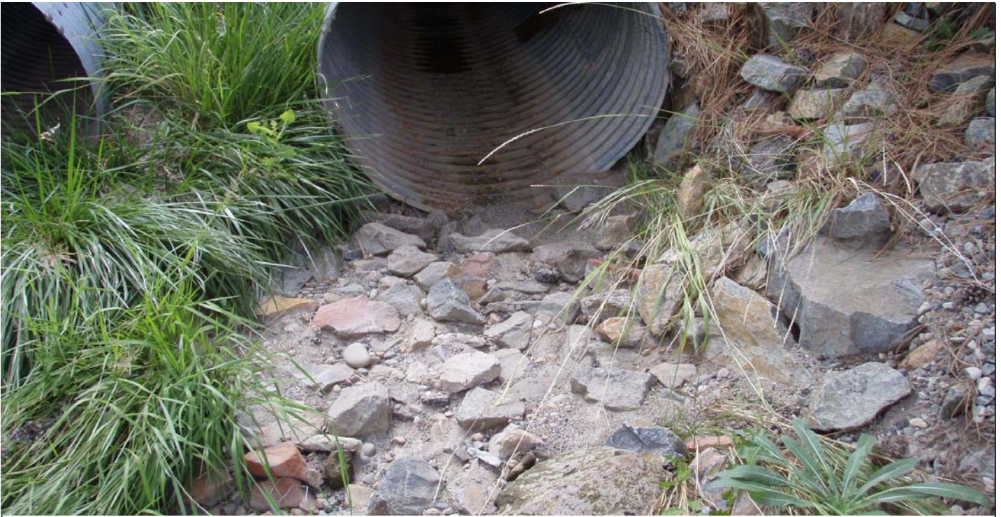
Photo 7600-2.JPG (taken 08/03/10) S00304060009 : Channel/Swale - Rip Rap.
