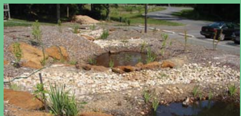
Regenerative Stormwater Conveyance
