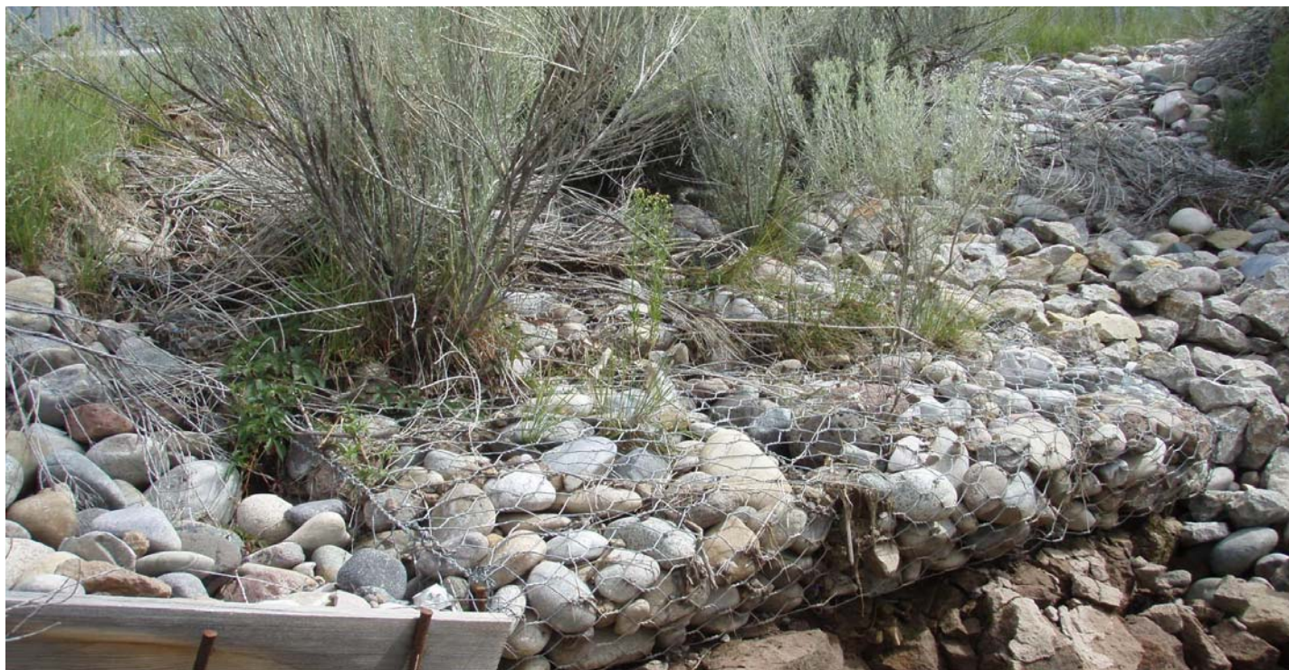
Photo 7600-6.JPG (taken 08/03/10) S00307020006 : Gabions - Gabion Blanket.
