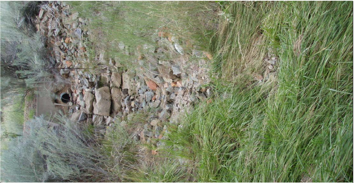
Photo 7600-4.JPG (taken 08/03/10) S00304060005 : Channel/Swale - Rip Rap.
