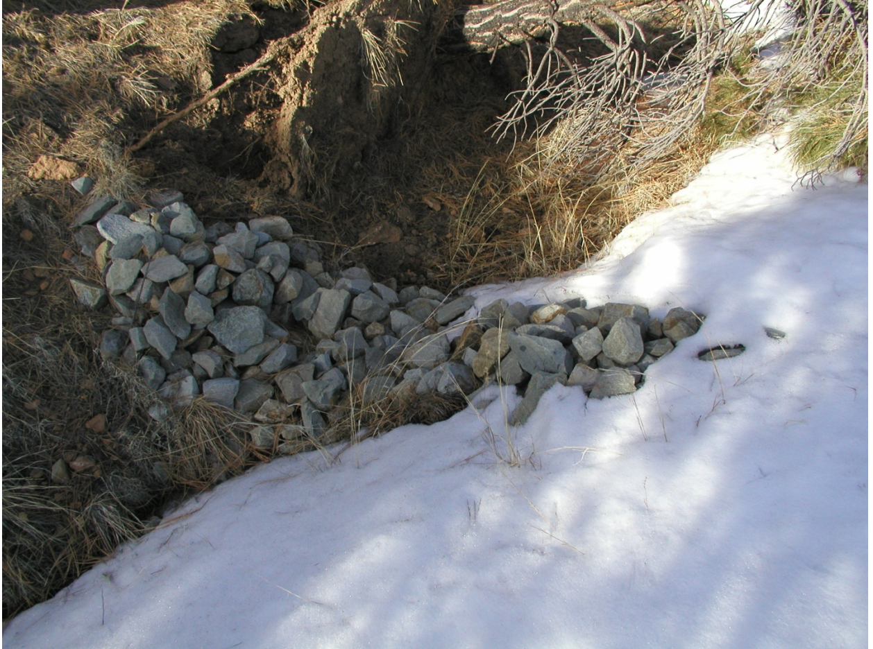
Figure 5 Repaired rock check dam
