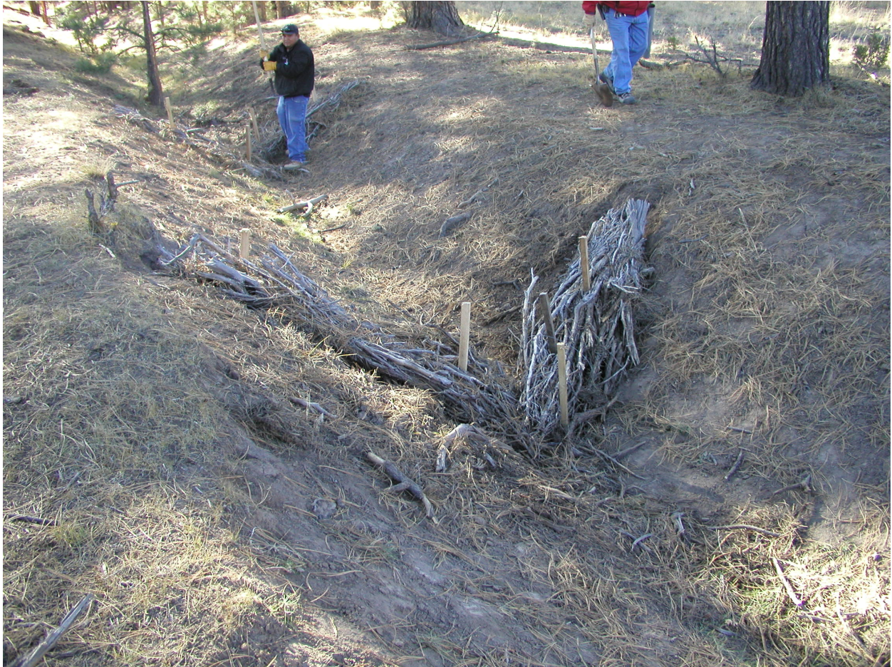
Figure 4 Juniper bale check dam in channel draining to 90s Line Pond repaired in November 2011
