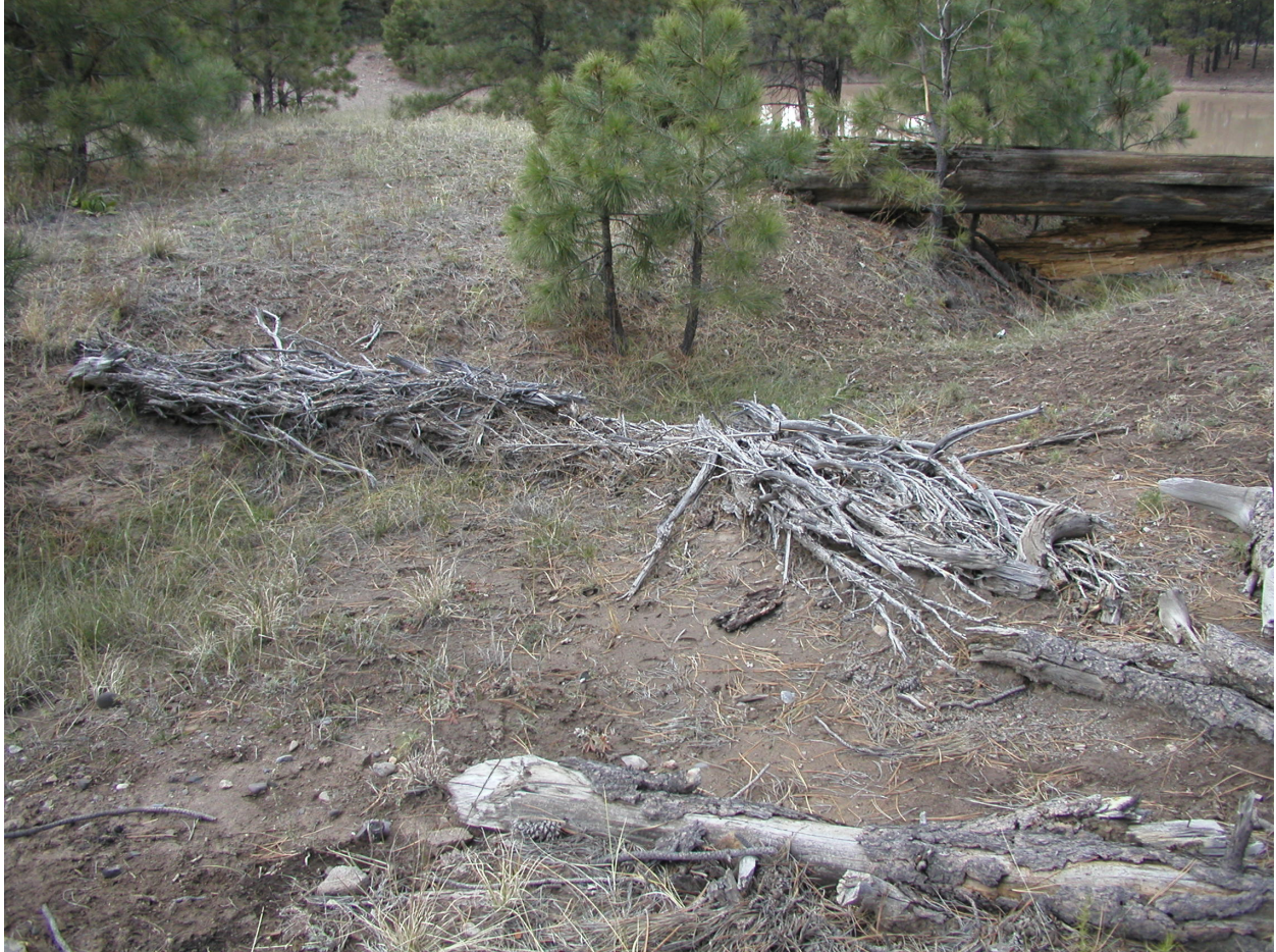
Figure 2 Juniper bale check dam in channel draining to 90s Line Pond
