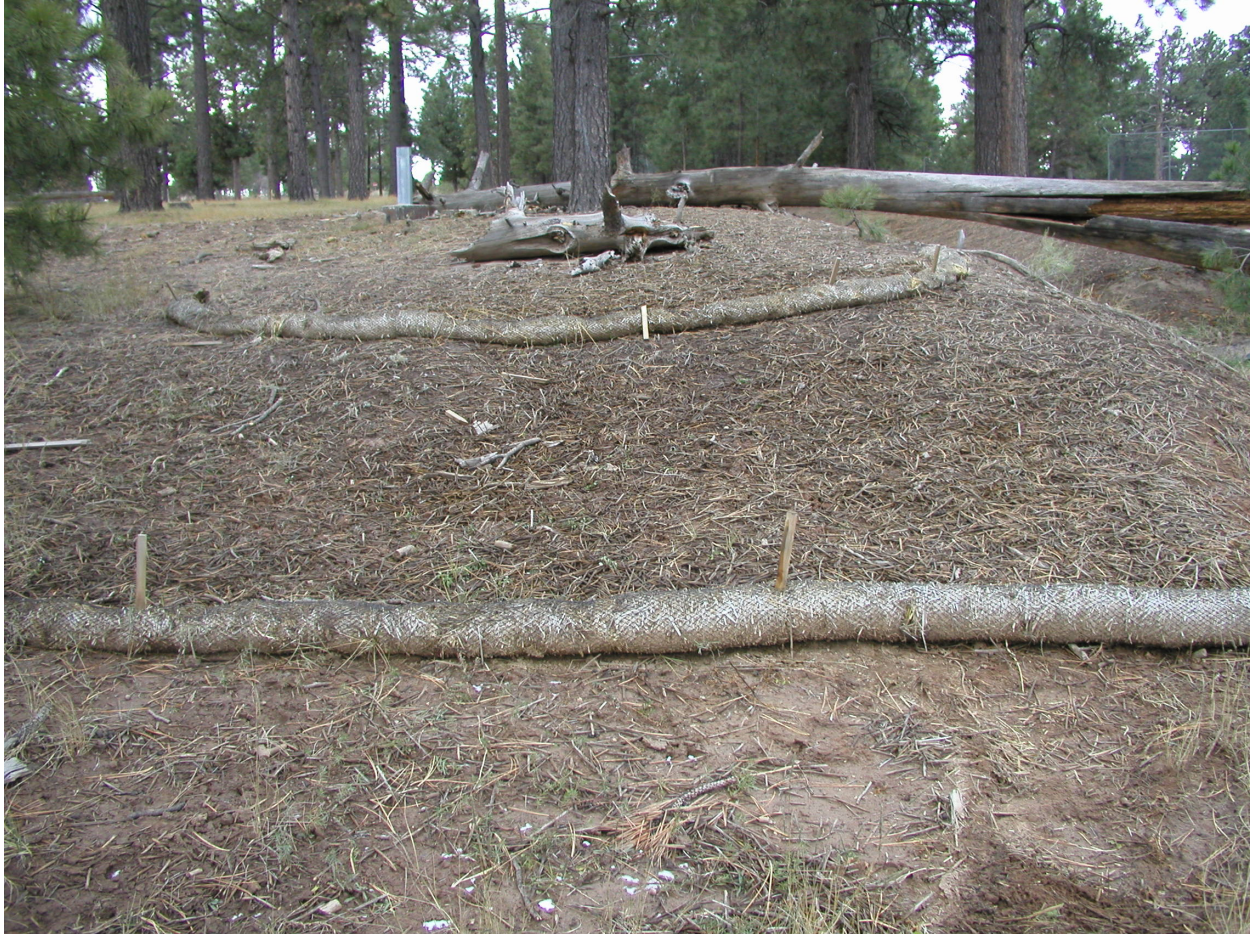
Figure 1 Seed, mulch, and straw wattles on bare slope draining to 90s Line Pond, November 2011
