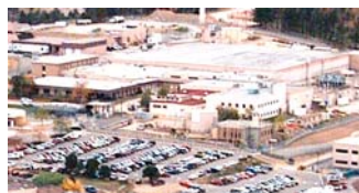
Plutonium Facility (TA-55)
