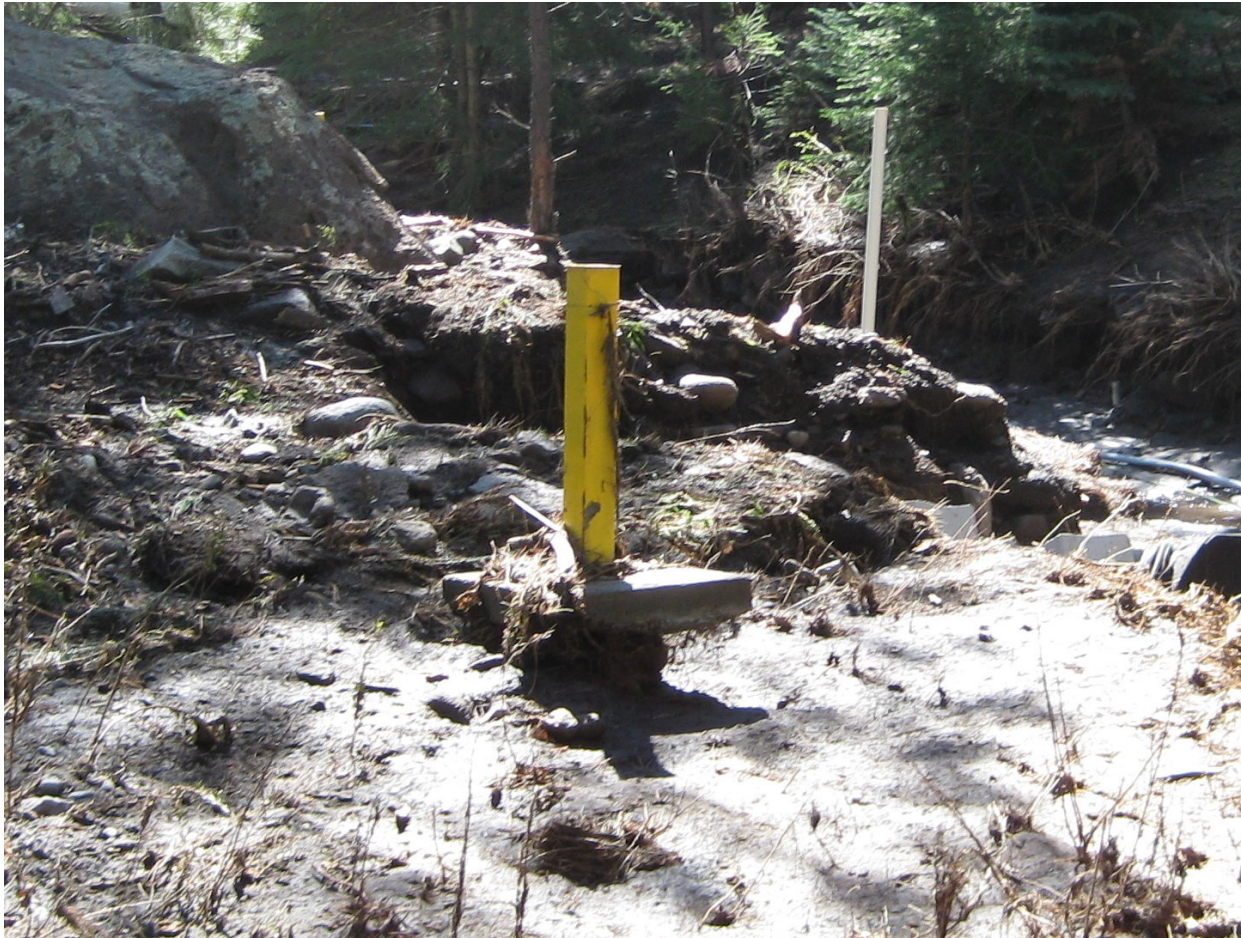
August 23, 2011: One of several upgradient alluvial wells compromised by flash flooding on 8/21/2011.
