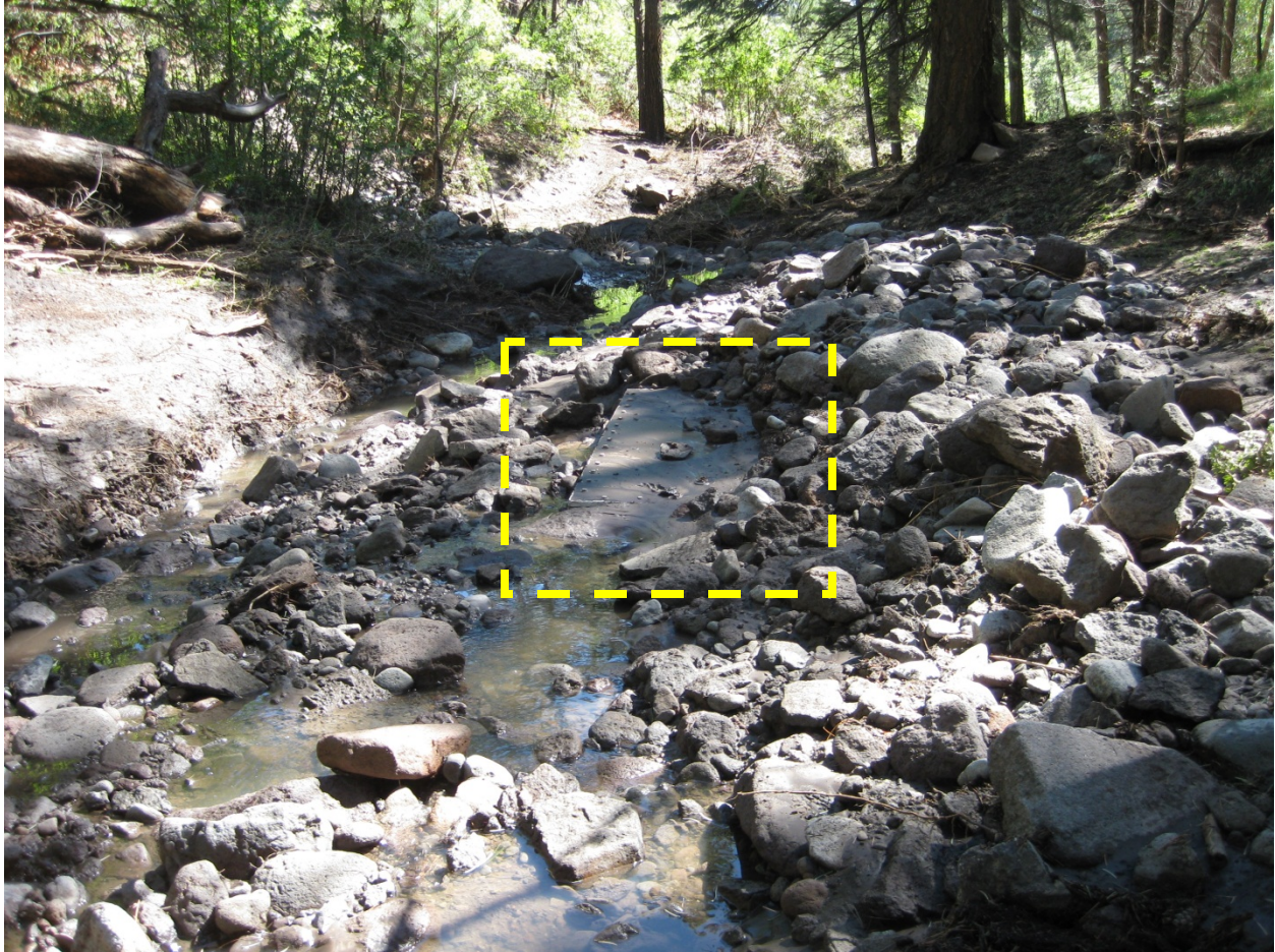
August 23, 2011: PRB vessel covered with sediment, rocks and debris in Cañon de Valle channel downgradient of PRB cutoff wall.
