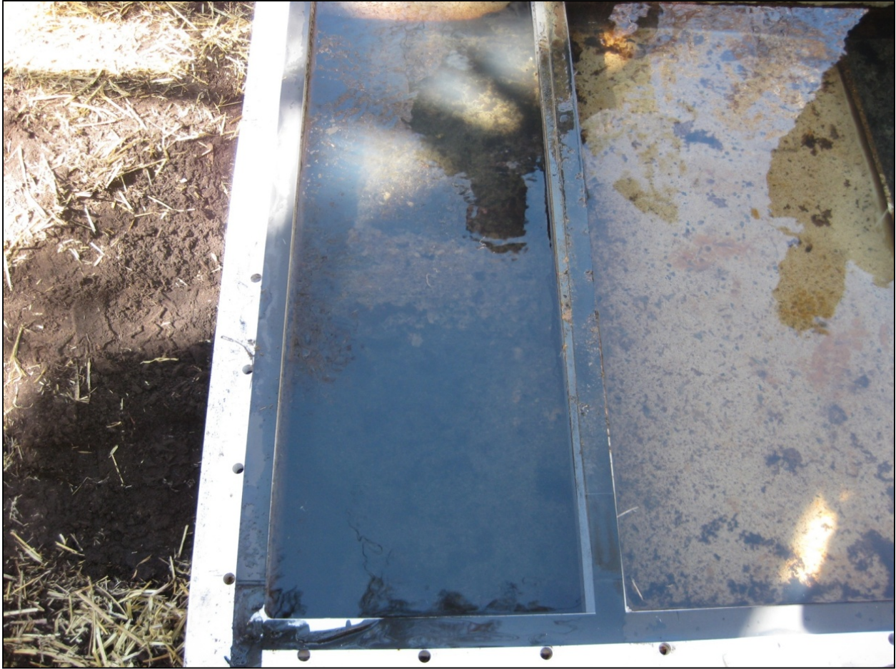
Figure 4.2-4 Water accumulation in the gravel and zeolite cells (March 23, 2011)
