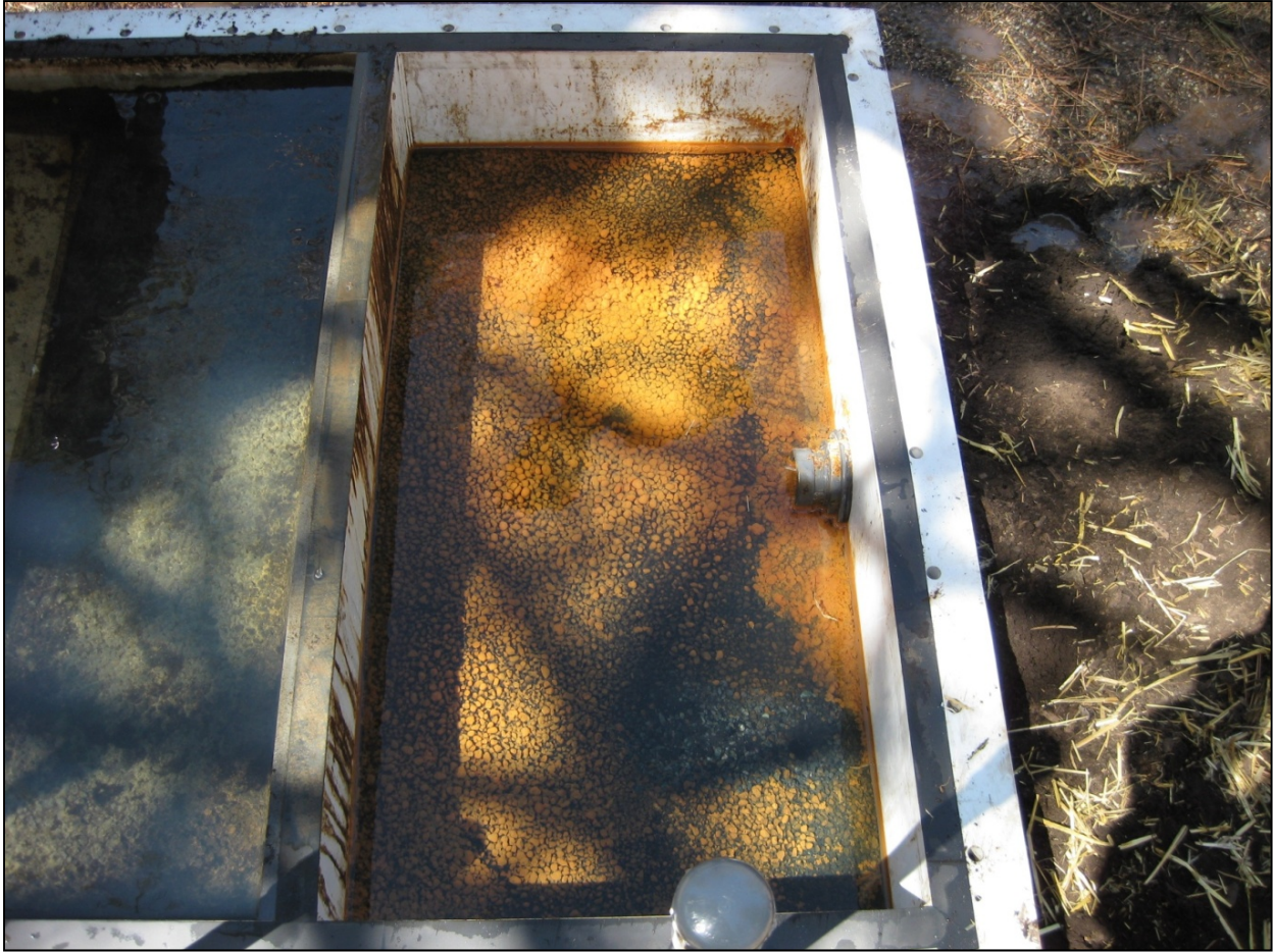
Figure 4.2-6 Impermeable ZVI material reduces flow/causes groundwater mounding in upgradient gravel cell
