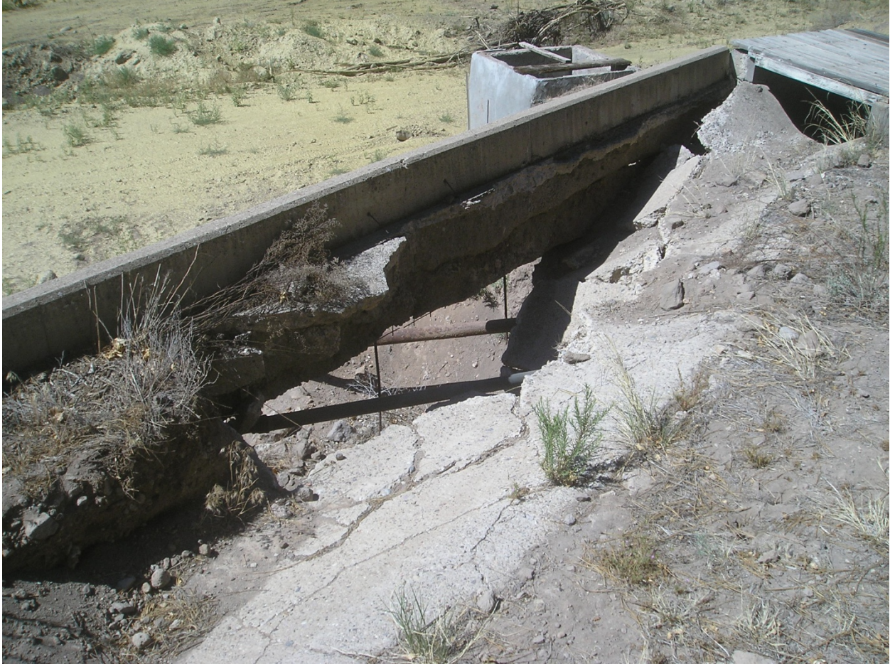
Figure 2 Photograph of the concrete trough at AOC 02-011(a)(i)
