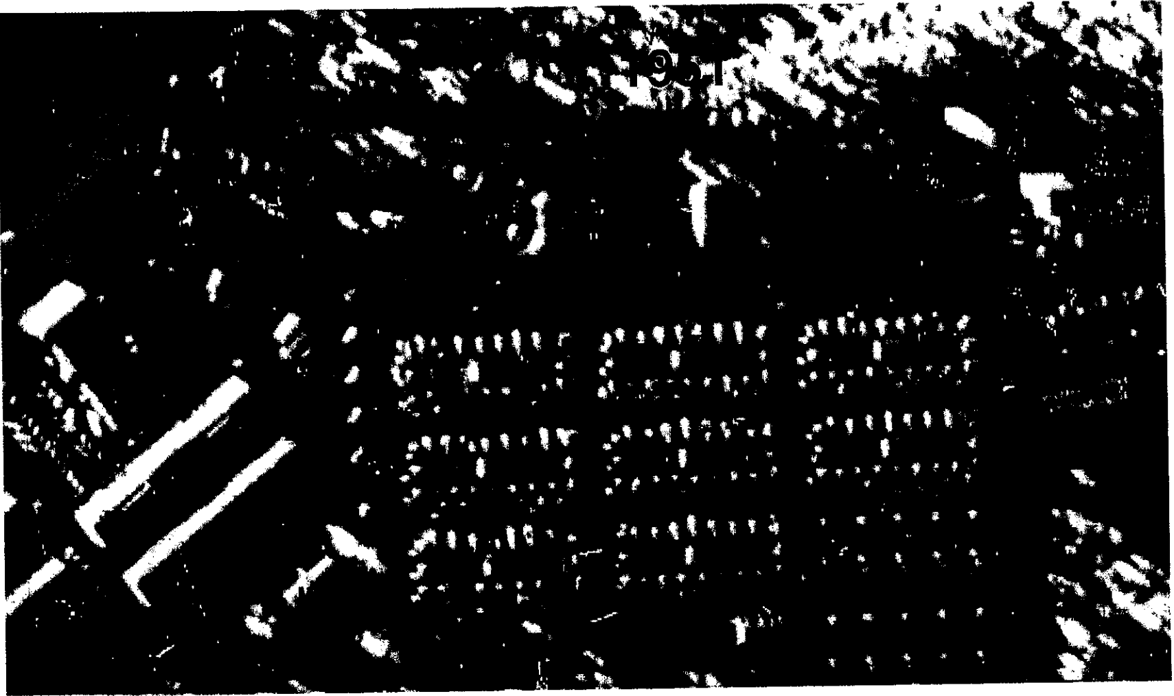
Figure 2.0-2. 1951 aerial photograph (negative)
