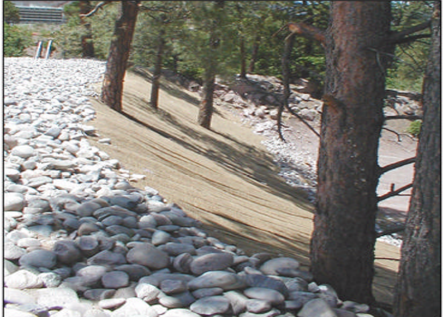
Potential Release Site 03-056(c) after cleanup activities
