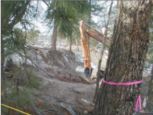
Excavation on slope at potential release site 03-056(c)
