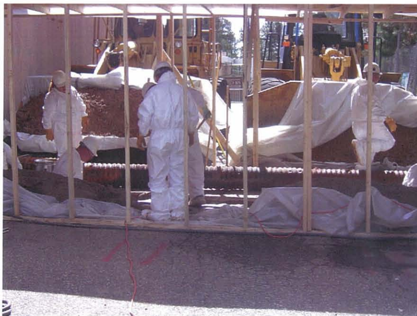
Photo 1. Removal of old culvert.
