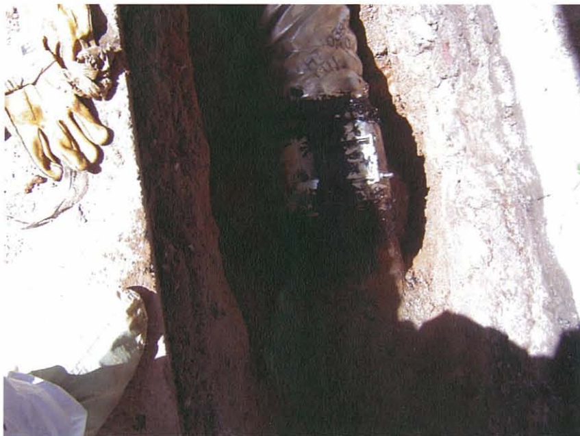
Photo 4. Mastic sealing of coupling.
