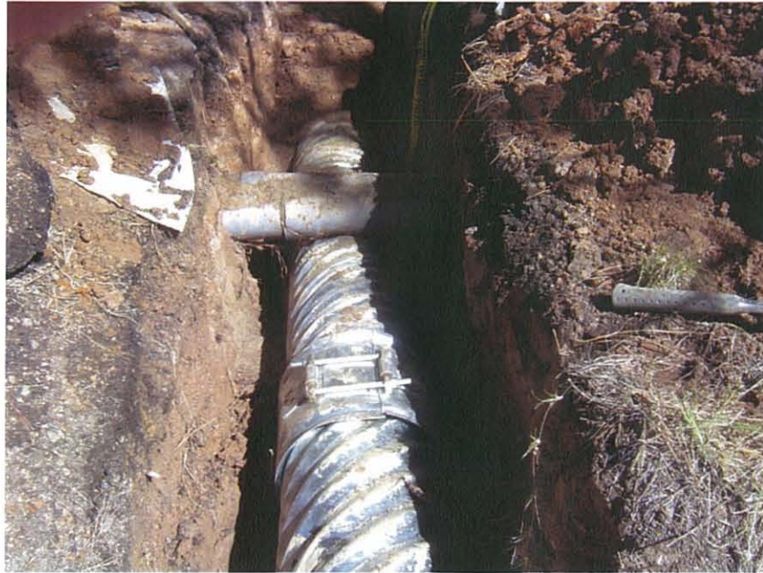
Photo 3. New CMP and existing utility line.
