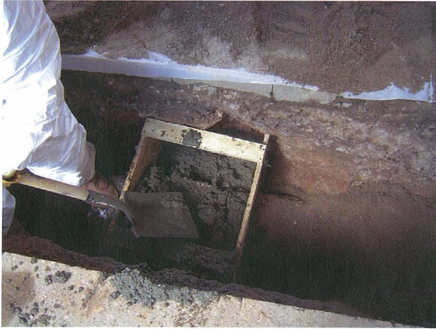
Photo 5. Encasing the coupling in concrete.
