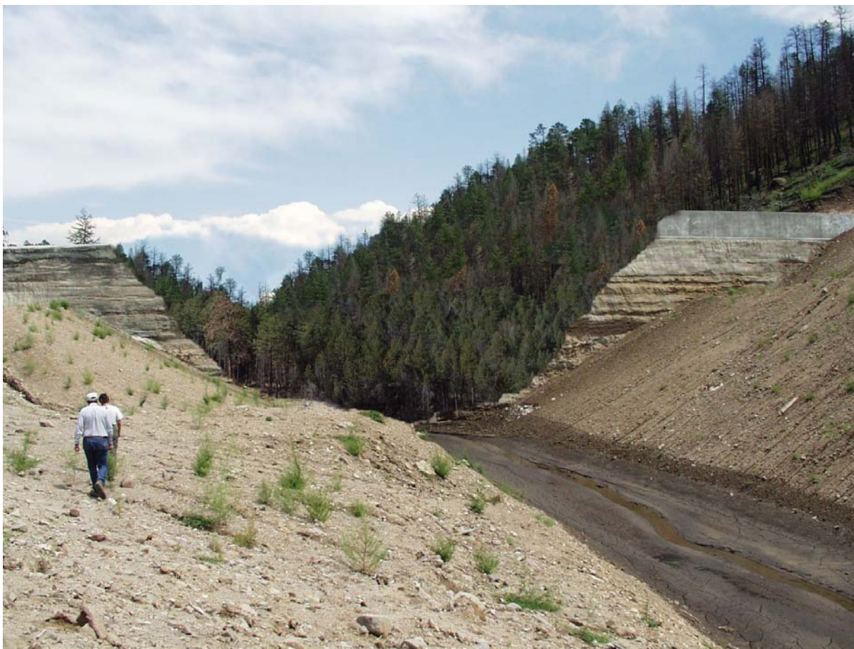
Figure 15. Digitally altered picture of the FRS to show partial removal.
