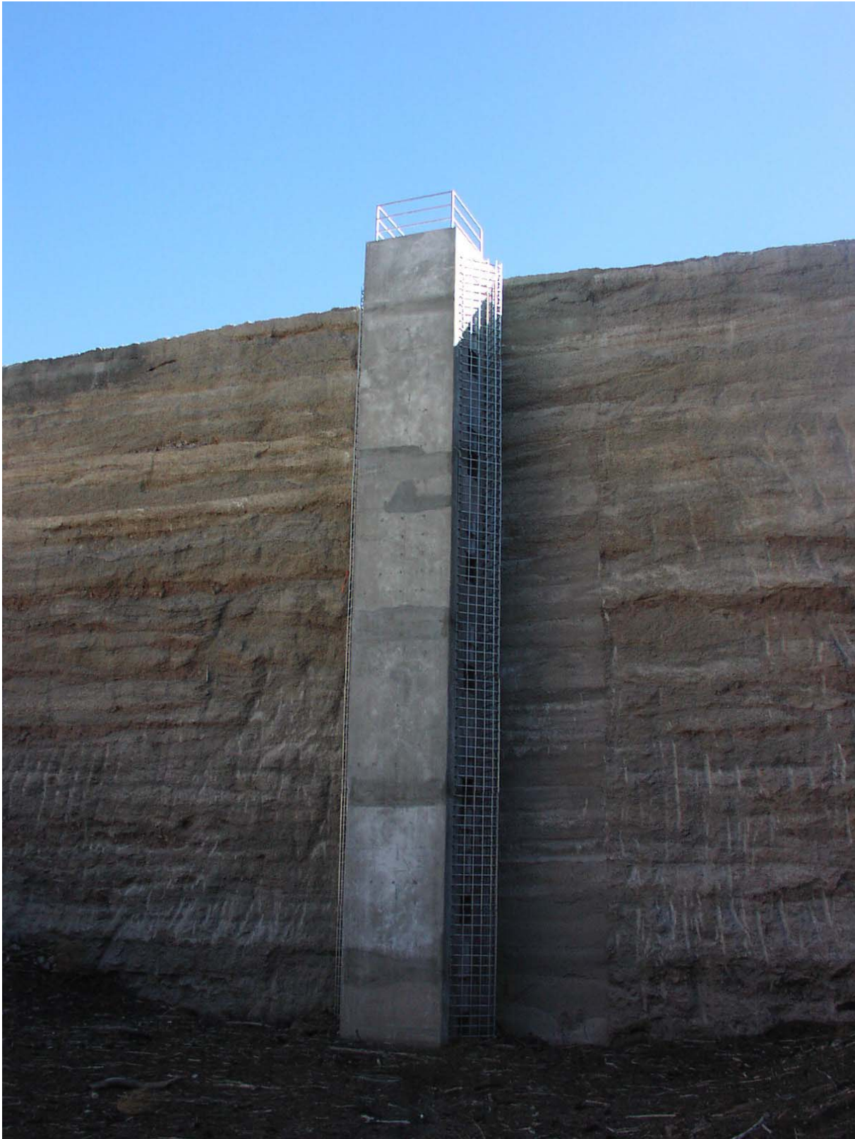
Figure 8. Close-up of the 73-ft (21.0-m) intake tower taken from reservoir on upstream side of FRS.
