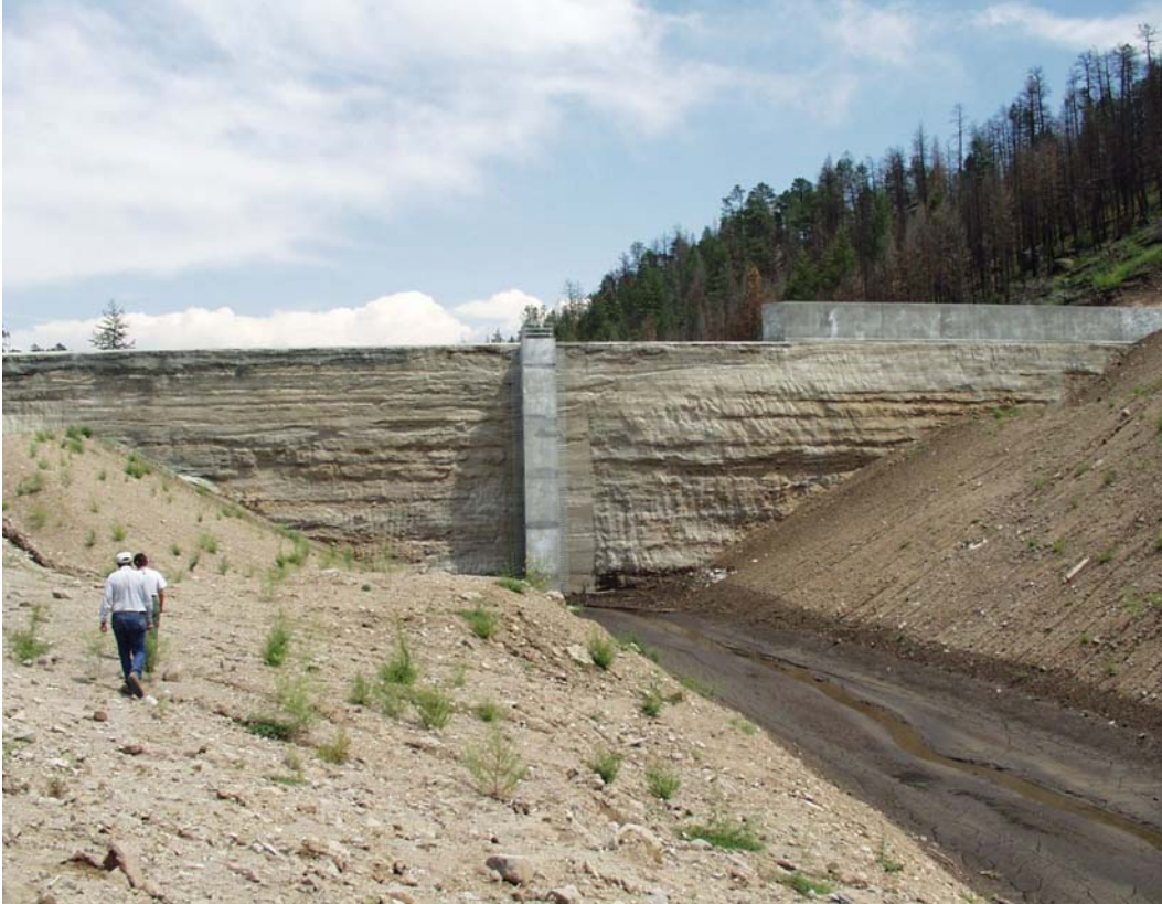
Figure 4. Upstream face of the FRS from upstream, north bank.
