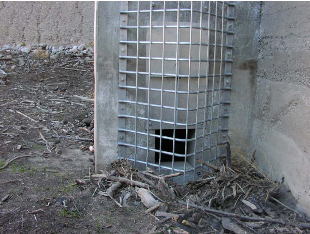
Figure 10. Close-up of inlet tower to show galvanized trash rack.
