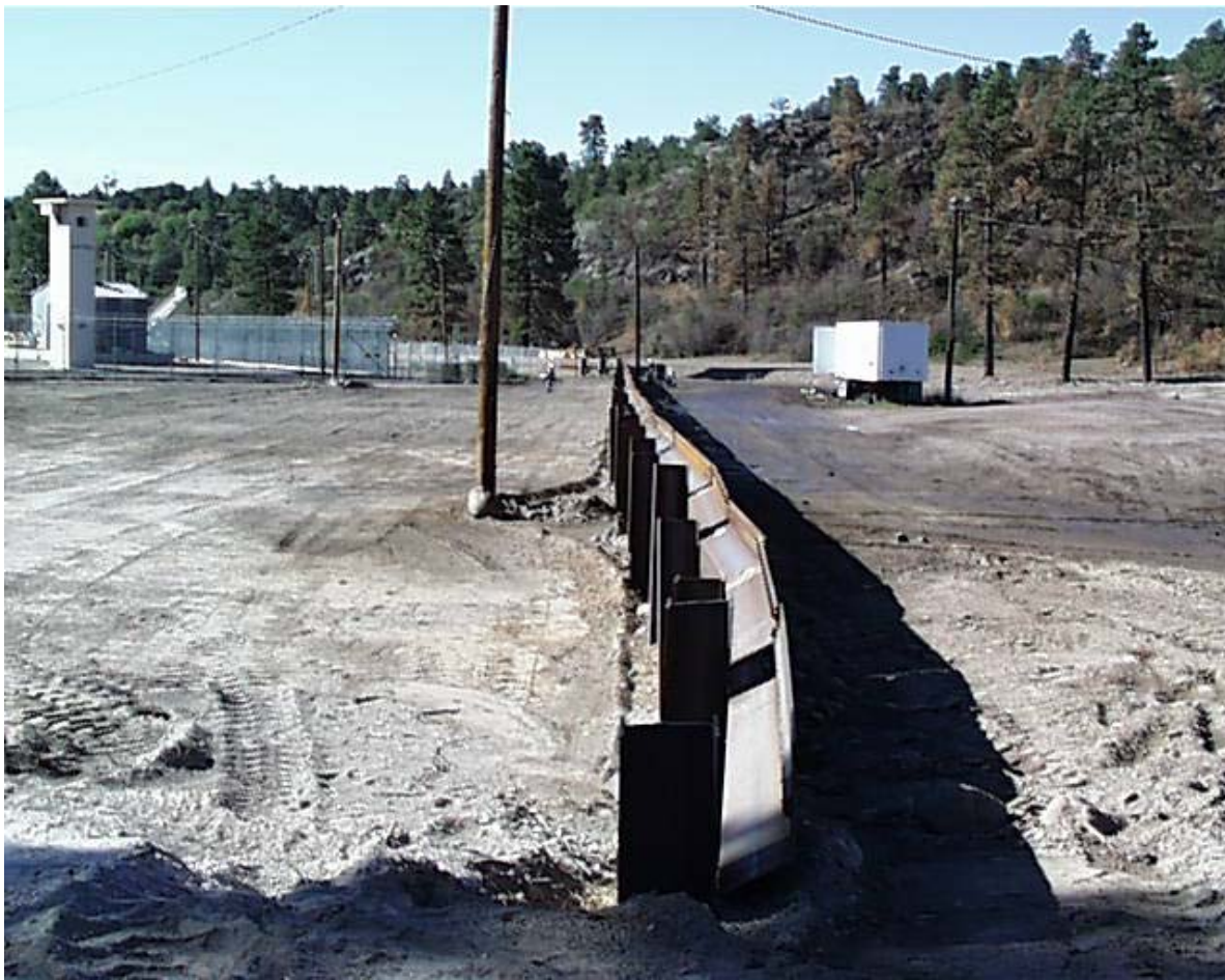
Figure 13. Steel diversion wall at TA-18 under construction.
